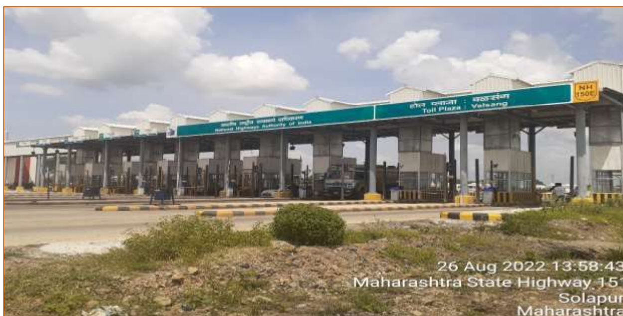
Figure 9-1 View of Valsang Toll Plaza
