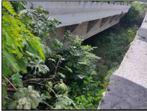
Minor Bridge at km. 66+020 (New Structure View)
