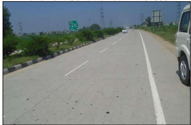
Rigid Pavement at km. 41+000
