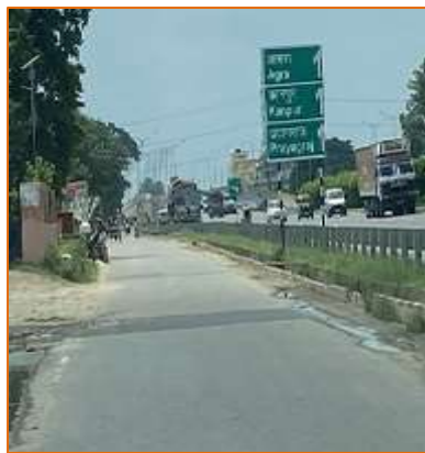
Slip Road at km. 764+700
