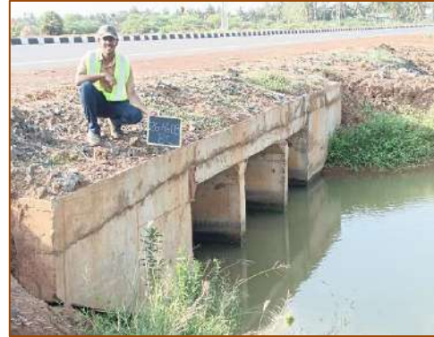
Box Culvert at km. 26+605
