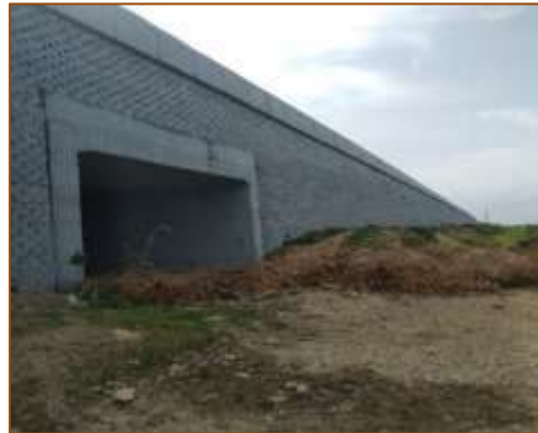
VUP at km. 393+695 (RHS)
