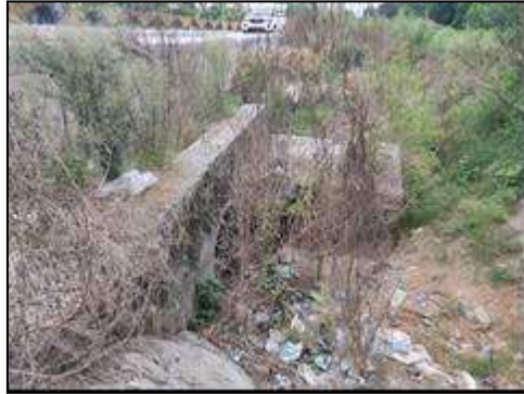
HP Culvert at km. 80+569
