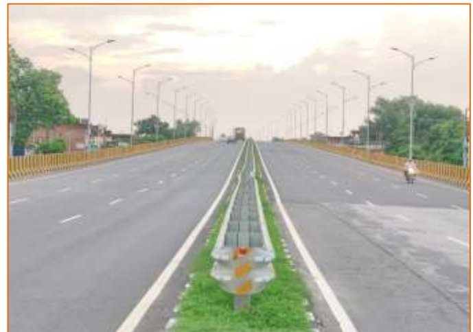
Highway Lighting at km. 740+300
