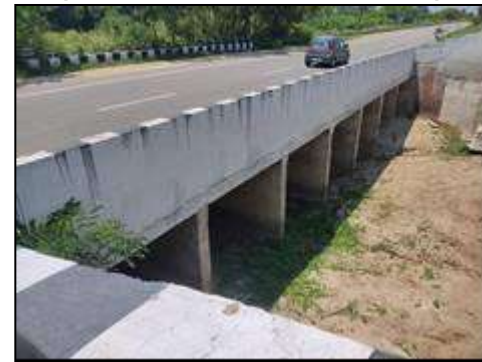
Minor Bridge at km. 57+981 (Existing Structure View)
