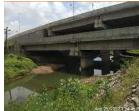
Side View of Minor Bridge at km. 117.796 - RHS (MCW & SR)
