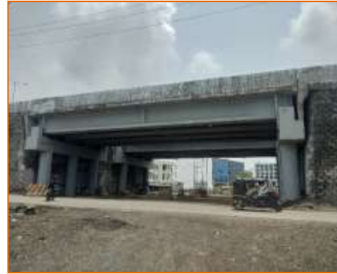
Side View of VUP at km. 58+570 (LHS)
