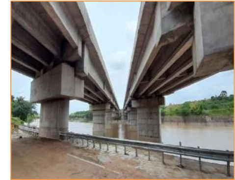
View of Major Bridge at km. 68+742
