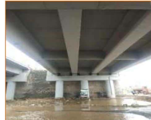
Bottom View of VUP at km. 12+420
