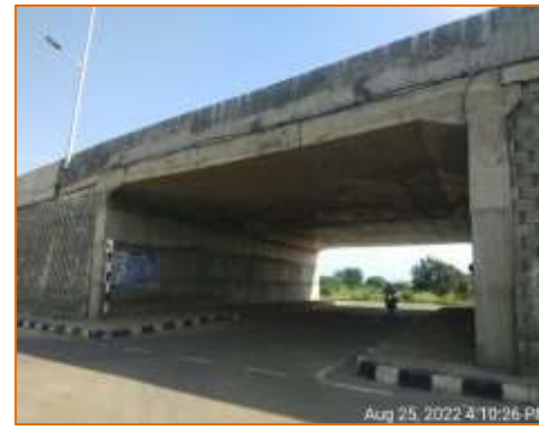
Side view of LVUP at km. 111.260 (RHS)
