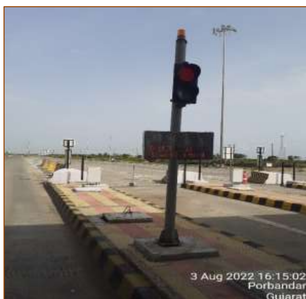
TP-1 at km. 409+500
