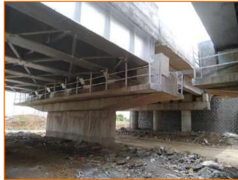
Rail Over Bridge at km. 294.125
