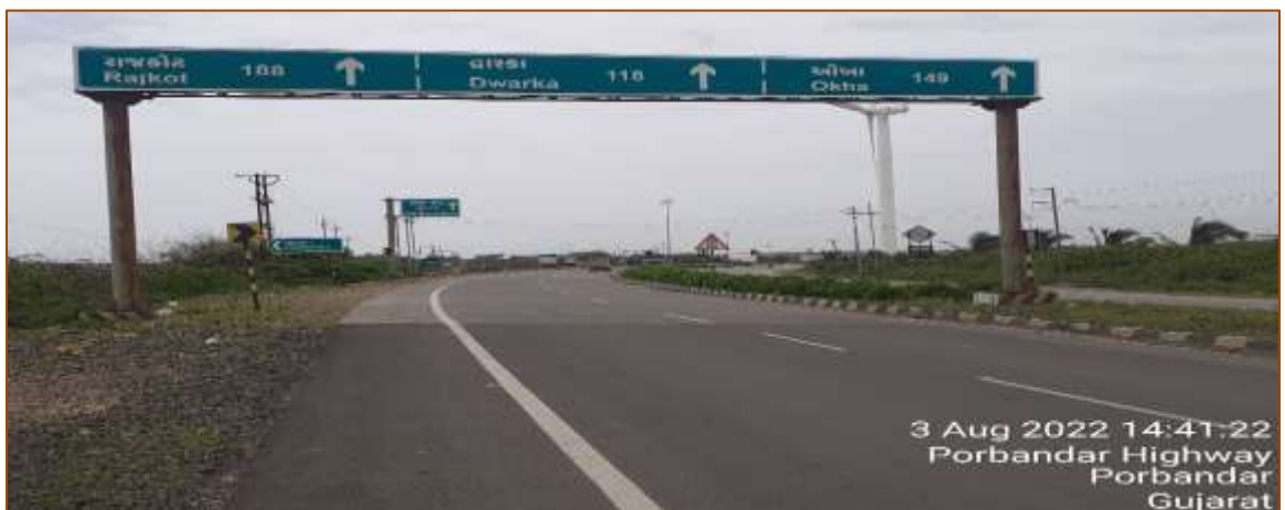
Figure 2-2 Start of project highway at km. 379+100
