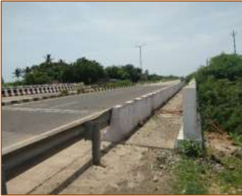
Minor Bridge at km. 427+321(RHS) - Widening - Wearing Coat
