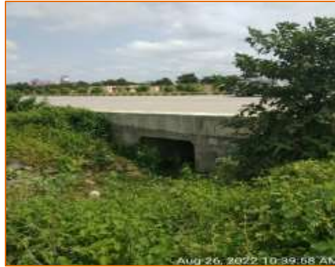
Box culvert at km. 125.495 - LHS (Reconstruction)
