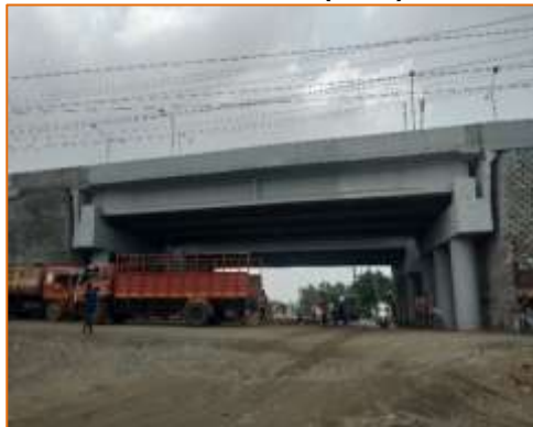
Side View of VUP at km. 55+300 (LHS)
