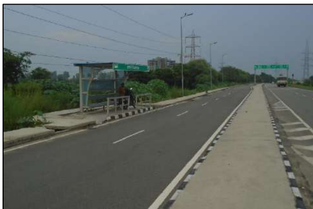
Bus Bay at km. 0+740
