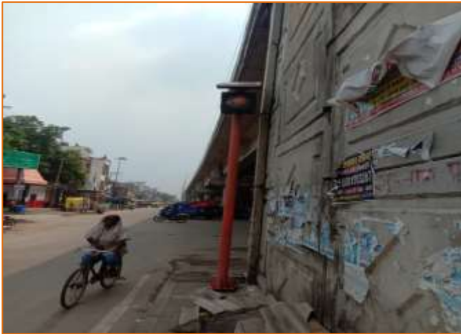
LED Blinker at km. 741+010
