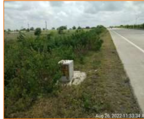
Pipe Culvert at km. 113.155 - RHS (Widening)
