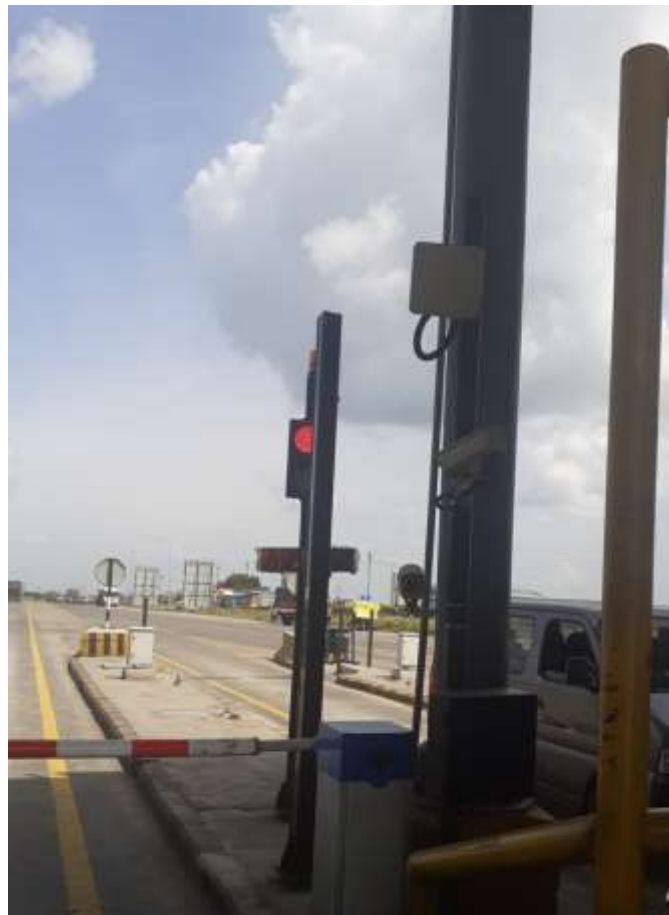
Figure 9-2 RFID ETC Reader mounted on Pole
