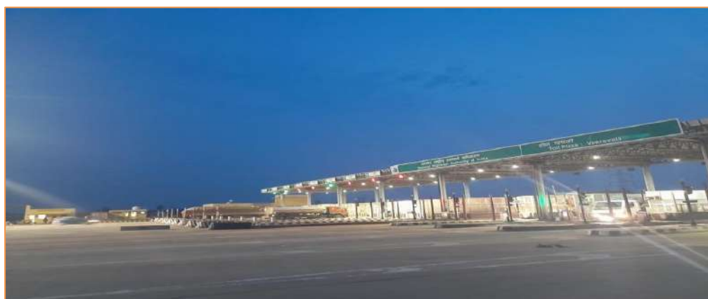
Figure 3-13 View of Toll Plaza
