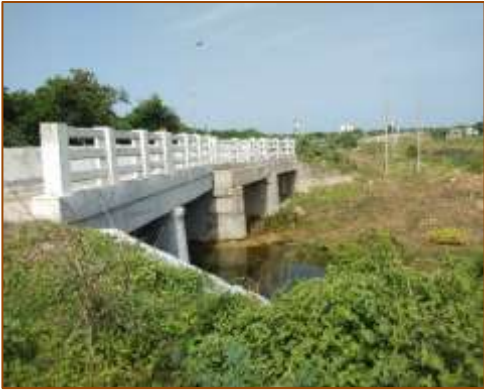
Side View of Minor Bridge at km. 483+502 (RHS) - Widening
