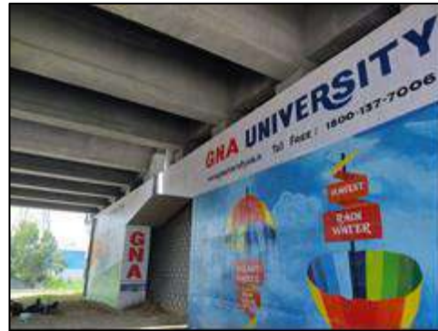
Flyover at km. 39+915
