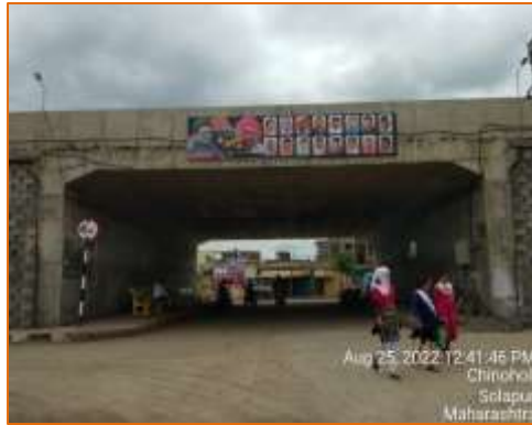
Side View of LVUP at km. 121.950 (RHS)
