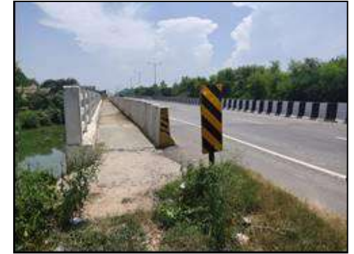
Minor Bridge at km 59+237 (top view)
