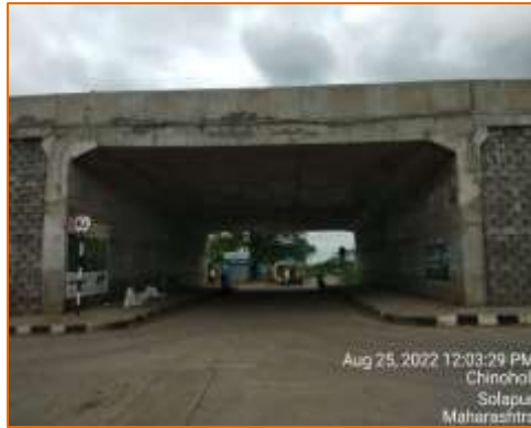
Side View of LVUP at km. 125.055 (RHS)
