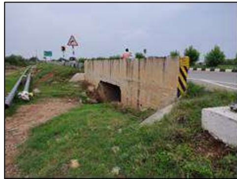
Box Culvert at km. 0+960
