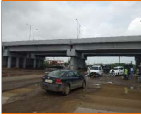
Side View of VUP at km. 12+420 (RHS)
