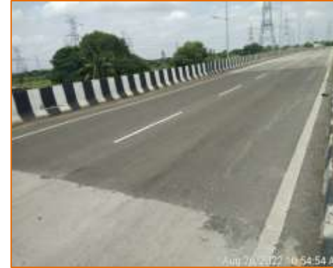
Good condition of BC surface of LVUP at km. 121.950 (LHS)
