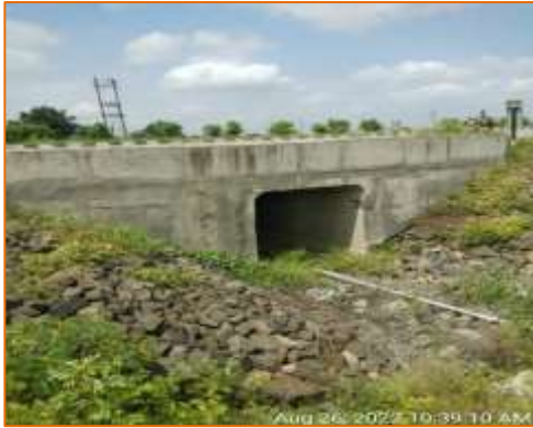
Box culvert at km. 125.495 - RHS (Reconstruction)
