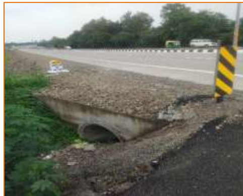
HPC at km. 66+010 (LHS)
