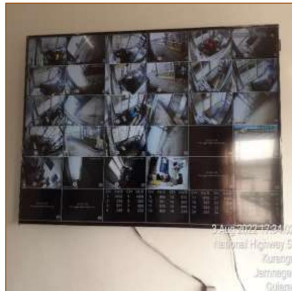
TP-2 at km. 470+875
