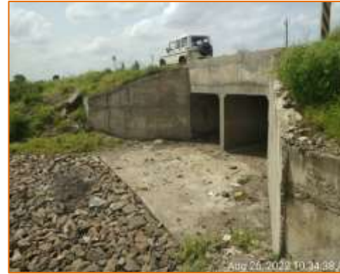
Box culvert at km. 126.643 - RHS (Reconstruction)
