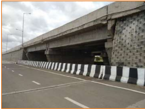
New Minor Bridge at km. 288.035
