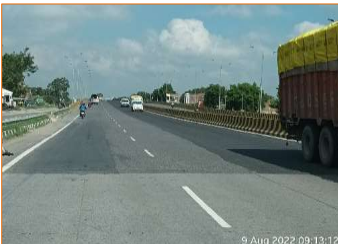
Road Marking to be done at km. 779+850
