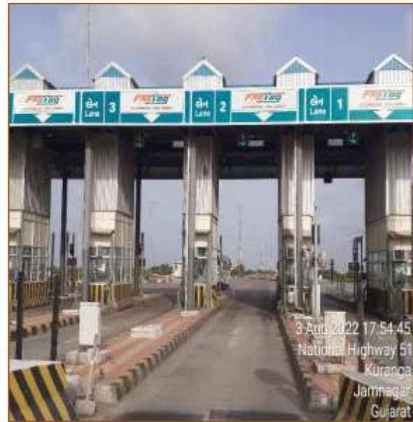
TP-2 at km. 470+875
