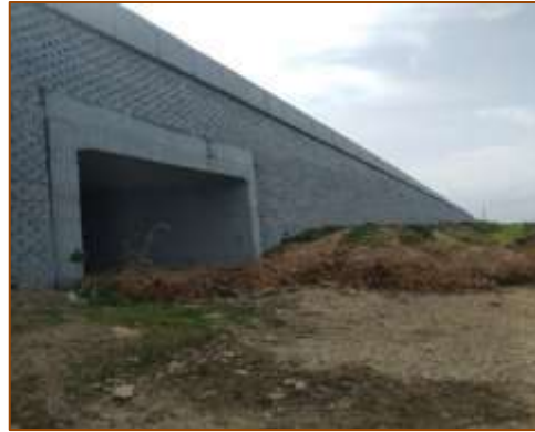
VUP at km. 393+695 (RHS)
