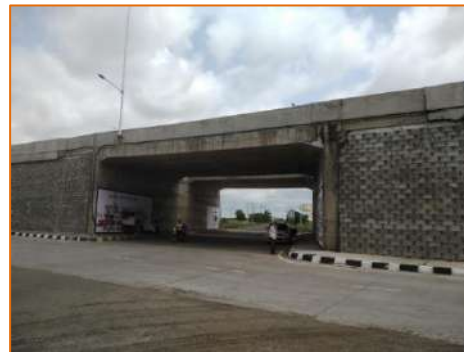
Vehicular Underpass at km. 292.758
