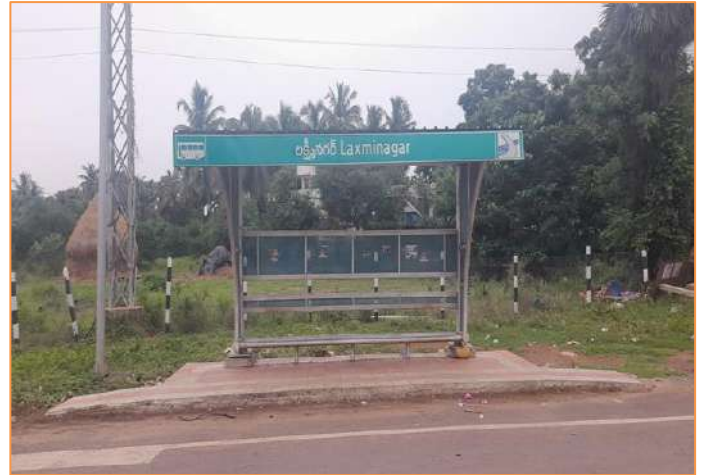
Bus Bay with Shelter at km. 56+140
