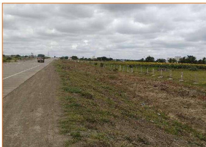
Avenue Plantation at km. 293+700
