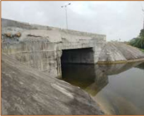
Side View of Minor Bridge at km. 460+812 (RHS) - New
