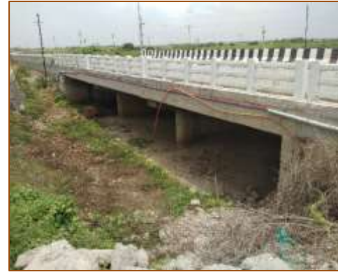
Side View of Minor Bridge at km. 449+894 (LHS) - New
