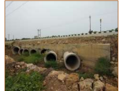
HPC at km. 456+200 (RHS)
