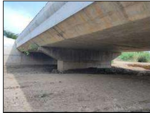
Minor Bridge at km. 68+519 (Substructure and Superstructure)
