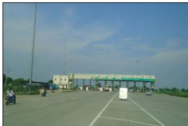
Behram Toll Plaza at km. 15+300
