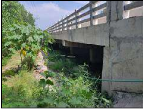
Minor Bridge at km. 64+791 (New Structure View)
