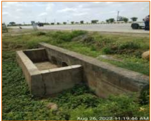
Pipe Culvert at km. 117.423 - RHS (Widening)
