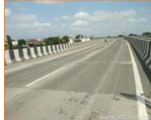
Good condition of BC surface of Flyover at km. 130.650 (LHS)
