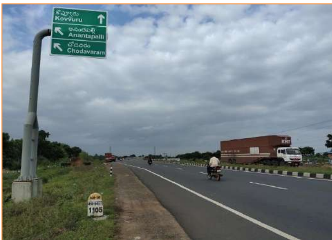
Cantilever Sign at km. 67+000
