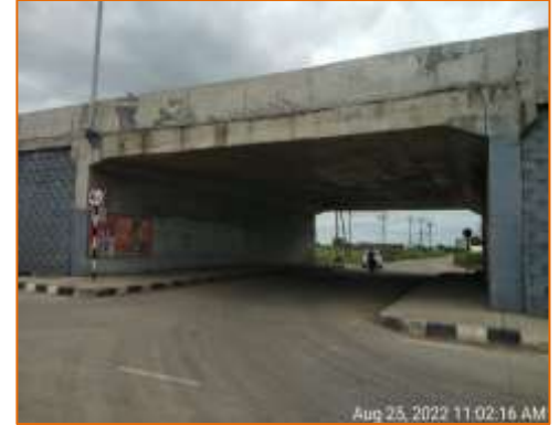
Side View of LVUP at km. 132.025 (RHS)
