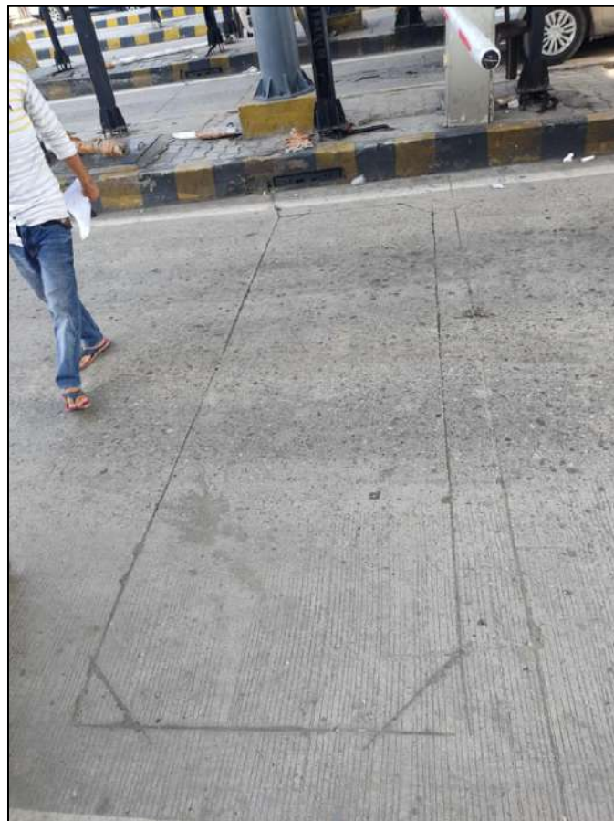
Figure 9-6 Inductive loop
