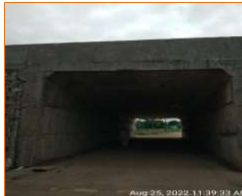
Side View of PUP at km. 130.485 - LHS (Under COS)
