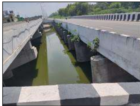
Major Bridge at km. 59+381 (Top View)
