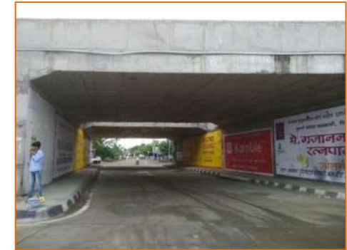
Light Vehicular Underpass at km. 298.613
