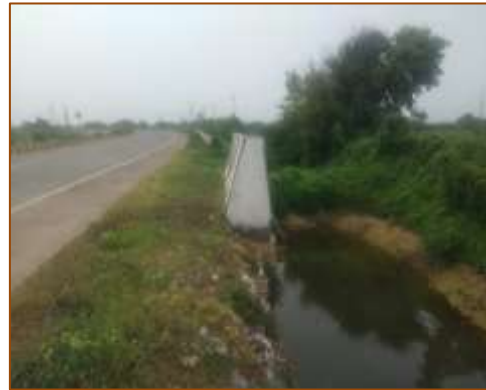
Slab culvert at km. 439+458 (RHS)
