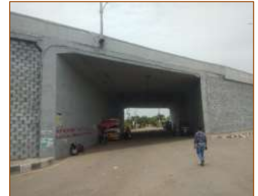
VUP at km. 432+050 (RHS) - Skew (Miyani) under COS
