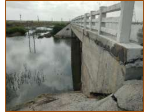
Side View of Minor Bridge at km. 492+030 (RHS) - New
