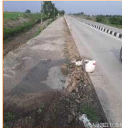
km. 46+000 single lane constructed
