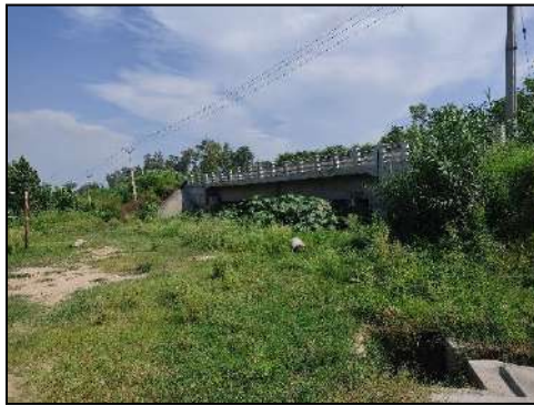
Minor Bridge at km. 62+704 (Existing Structure View)
