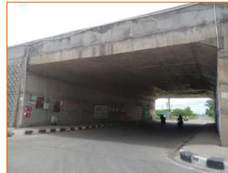
Light Vehicular Underpass at km. 285.432
