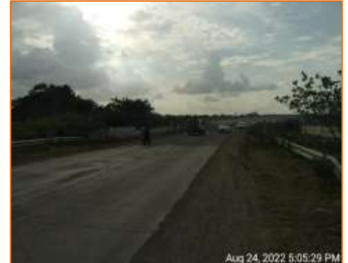
View of MNB at km. 99.586 (LHS)
