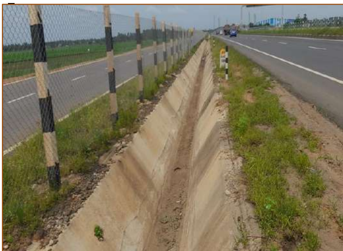
V Drain at km. 78+900
