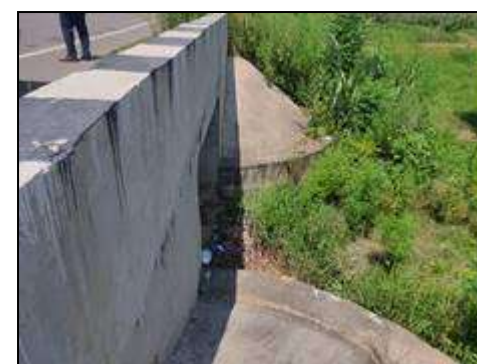
Box Culvert at km. 48+800
