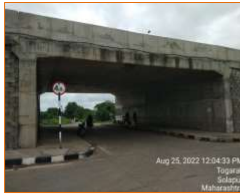
Side View of LVUP at km. 125.055 (LHS)
