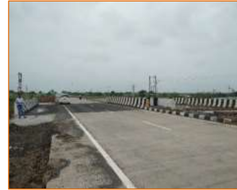
Wearing Coat of Minor Bridge at km. 13+410 (LHS)
