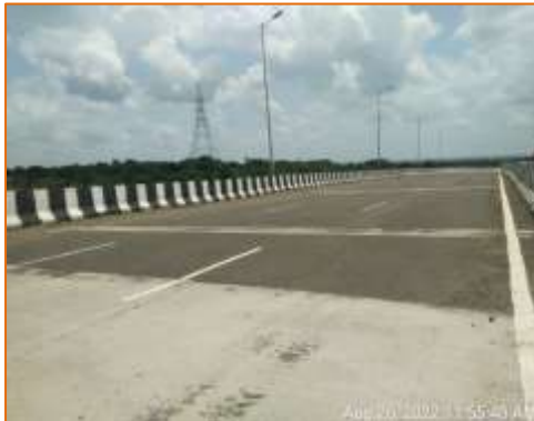
Flyover at km. 106.240 (RHS)
