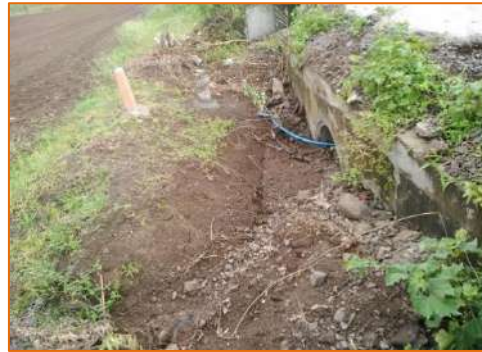
Pipe Culvert at km. 299+507
