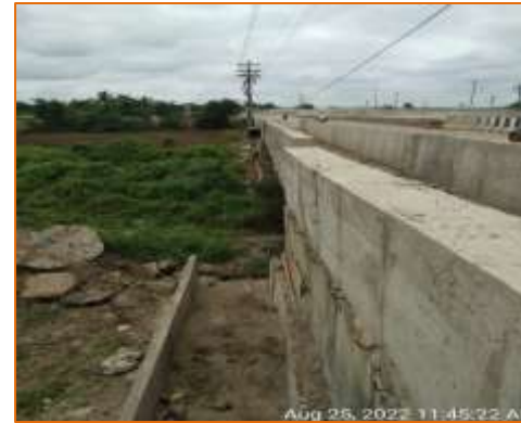
Side View of Minor Bridge at km. 130.149 - RHS (Not accessible)
