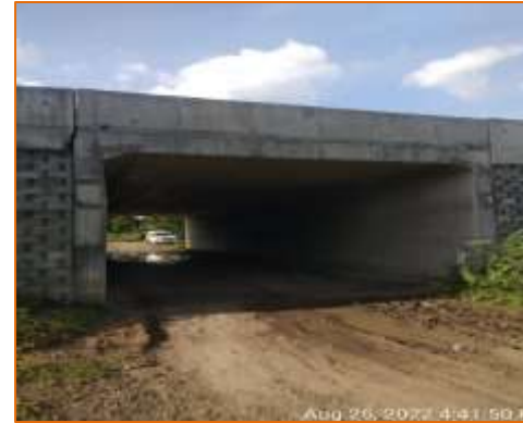
Side View of PUP at km. 104.820 (LHS) - Under COS
