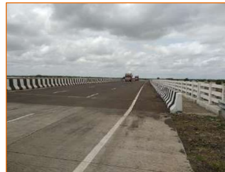
New Major Bridge at km. 280.420
