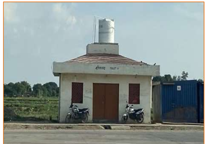
Toilet Block at Toll Plaza
