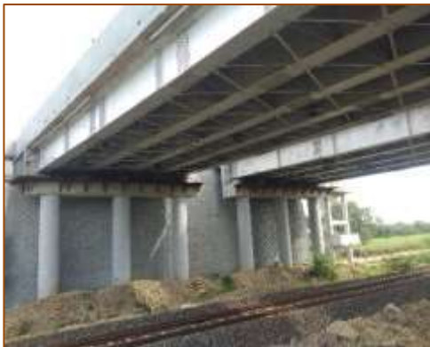
Side View of ROB at km. 393+642 (RHS)
