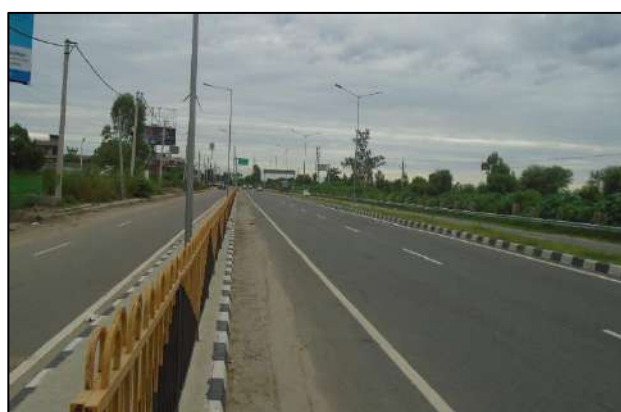
Approach to End of Project Road
