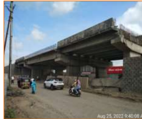
Side View of Flyover at km. 136.857 (LHS)
