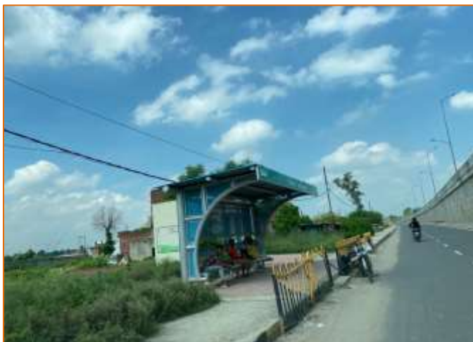
Bus Shelter at km. 775 + 900
