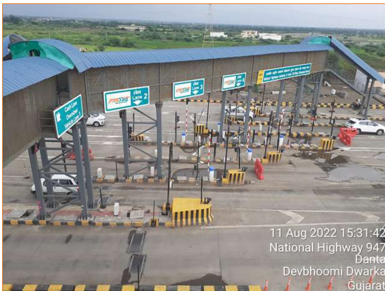
Figure 8-1 Views of Dharampur Dante Toll Plaza
