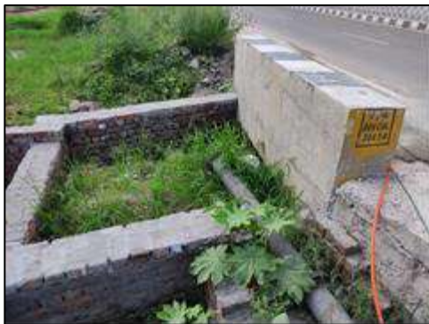
Box Culvert at km. 6+650
