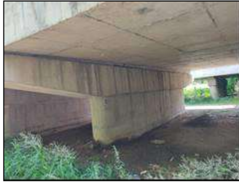
Minor Bridge at km. 64+791 (Existing Structure inner View)
