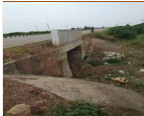
Slab culvert at km. 444+062 (RHS)
