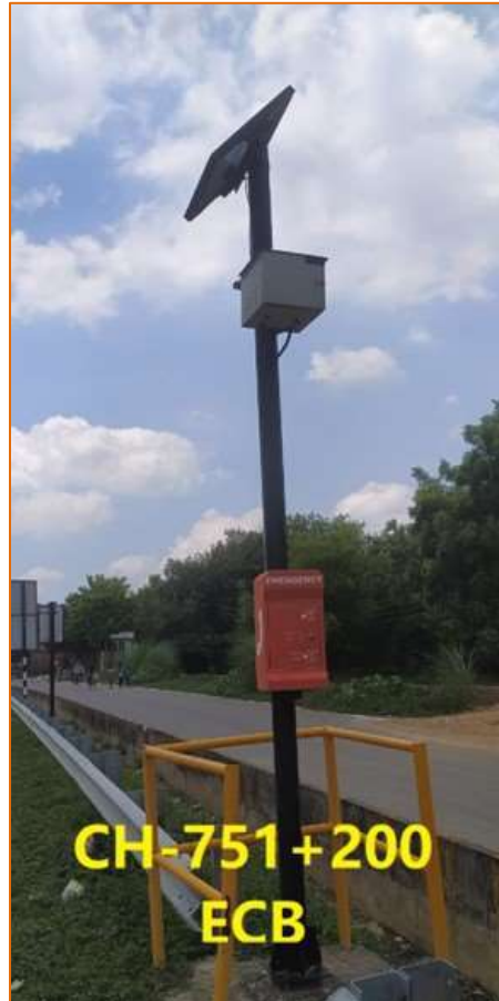
Figure 9-6 ECB at km. 751.200
