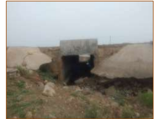
Slab culvert at km. 441+648 (RHS)
