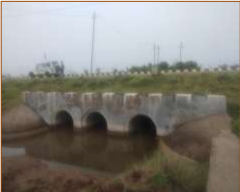
HPC at km. 437+025 (LHS)
