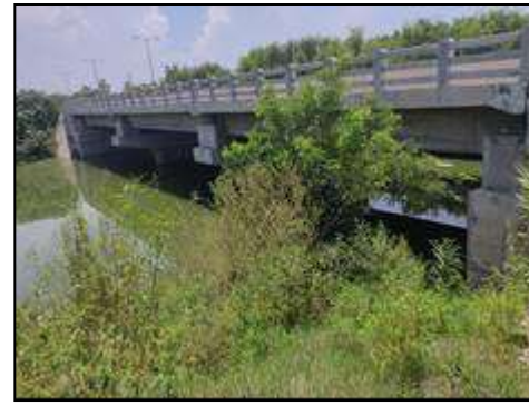
Minor Bridge at km 59+237 (New Structure View)
