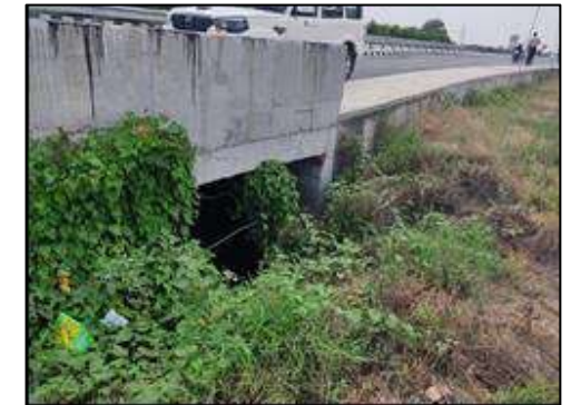
Box Culvert at km. 6+068
