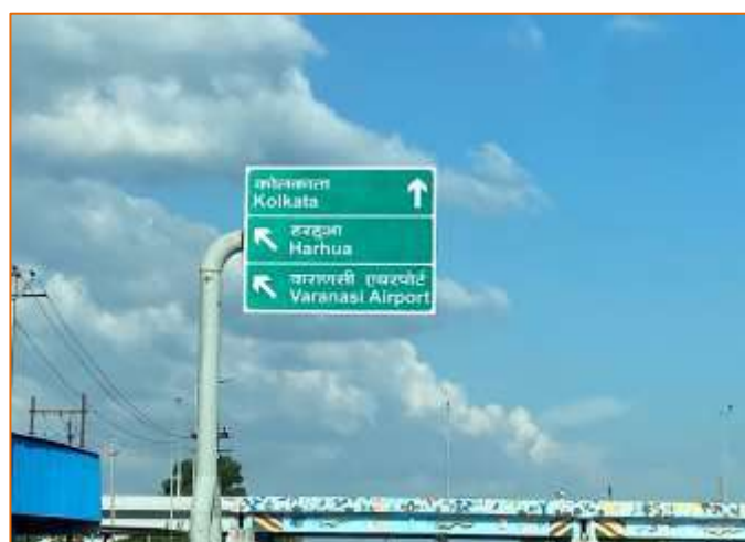
Cantilever Gantry Sign at km. 782+500
