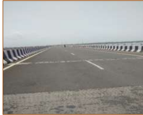
Major Bridge - km. 433+295 (LHS) Wearing Coat
