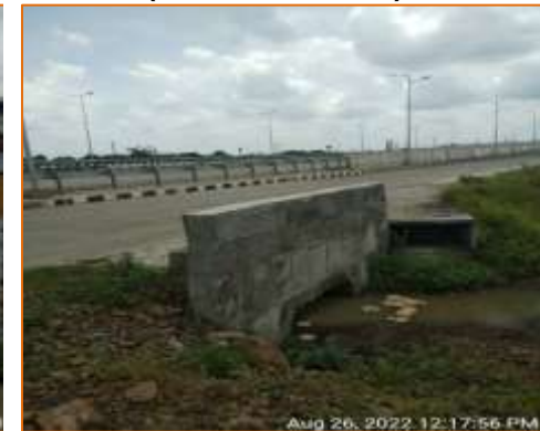
Box culvert at km. 133.524 - LHS (Reconstruction)
