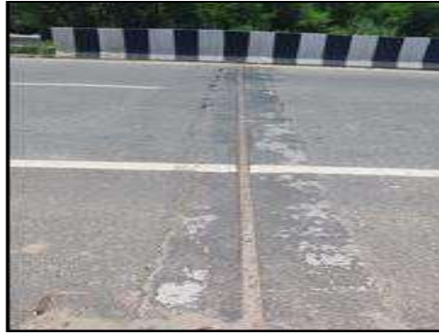
Minor Bridge at km 59+237 (Expansion Joint)
