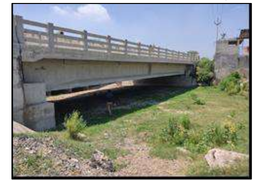
Minor Bridge at km. 57+981 (New Structure View)
