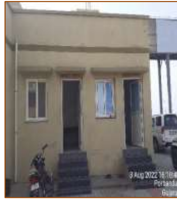
Highway Aid / Medical Room
