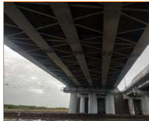
Bottom View of ROB's Girders at km. 0+527
