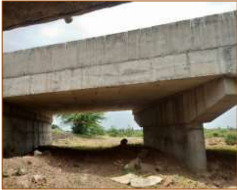
Bottom of Minor Bridge at km. 449+894 (LHS) - New
