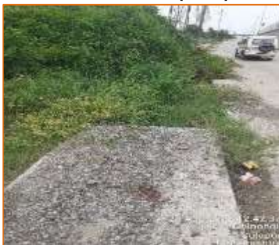
km. 121.470 (RHS) partially completed
