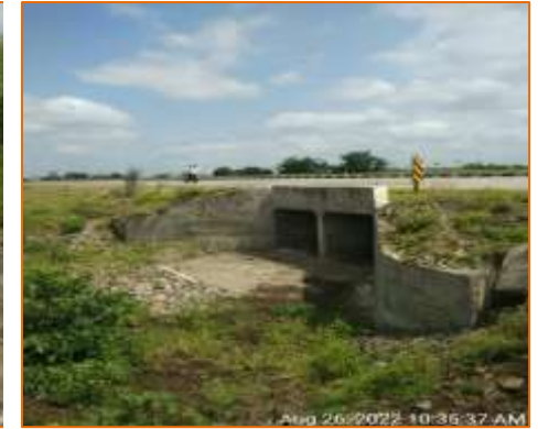
Box culvert at km. 126.643 - LHS (Reconstruction)
