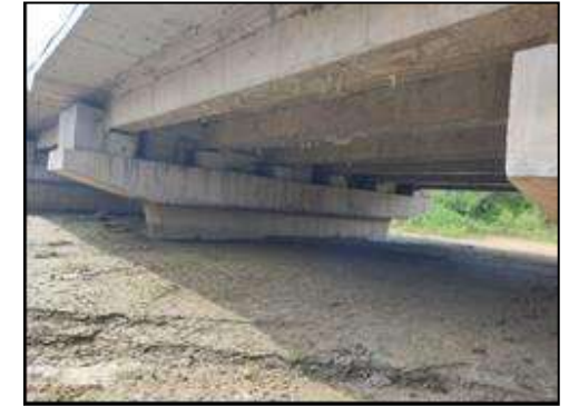
Minor Bridge at km. 68+519 (Substructure and Super structure)
