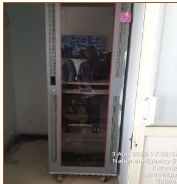
TP-2 at km. 470+875
