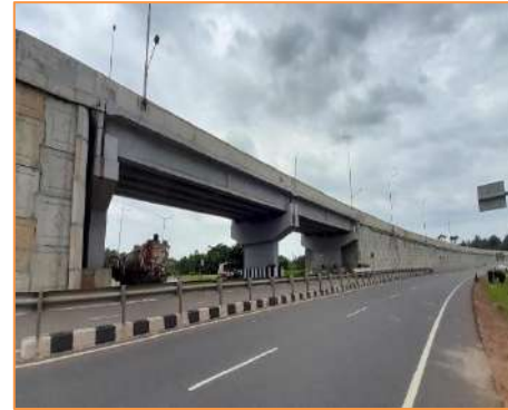
View of UDFO at km. 34+915
