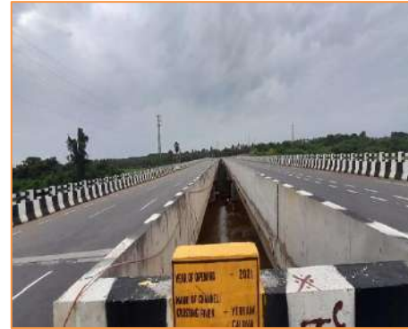
View of Major Bridge at km. 51+929
