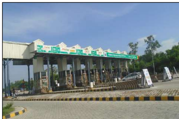
Bachhwan Toll Plaza at km. 70+240
