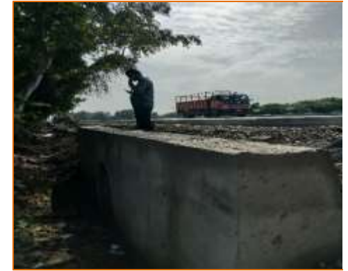
HPC at km. 32+520 (LHS)
