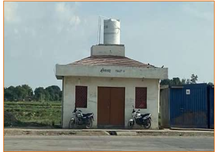
Toilet Block at Toll Plaza
