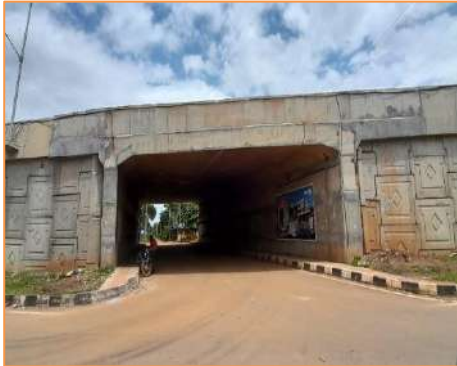
View of LVUP at km 27+790
