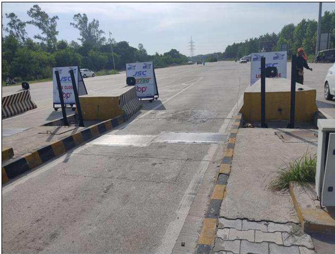
Figure 9-12 Medium Speed Weigh in Motion (MSWIM)
