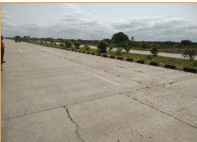
Panel Repair work done at km. 276+050 (LHS)
