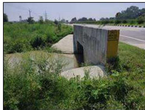
Box Culvert at km. 37+480
