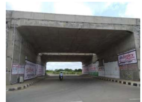
Vehicular Underpass at km. 287.300
