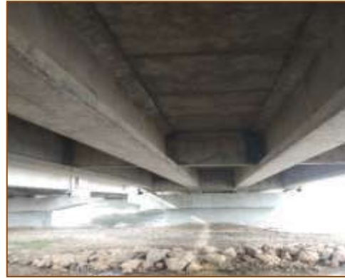
Bottom View of MJB Girder at km. 386+750 (RHS)
