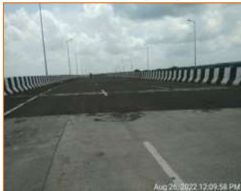
BC surface of Flyover at km. 102.700 (RHS)
