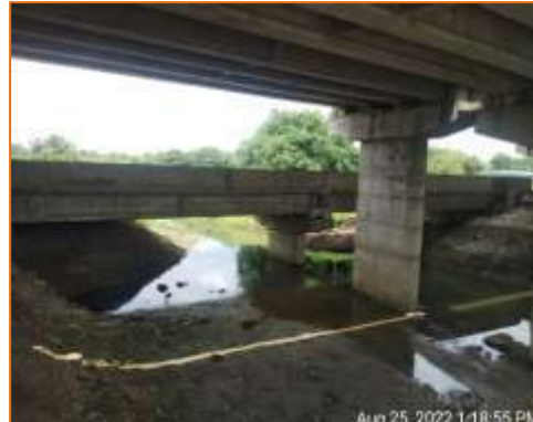
Bottom & side view of Minor Bridge at km. 117.796 (RHS)
