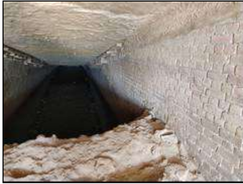
Minor Bridge at km. 57+981 (Existing Structure Inner View)
