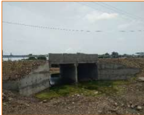
Side View of Minor Bridge at km. 64+660 (LHS)
