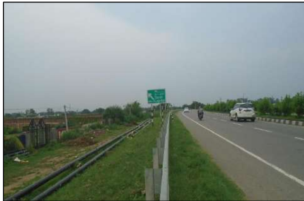
Crash Barrier at high embankment
