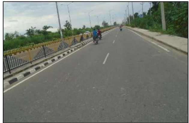
Pedestrian Guard Rail at km. 69+400
