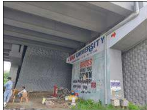
Flyover at km. 4+225
