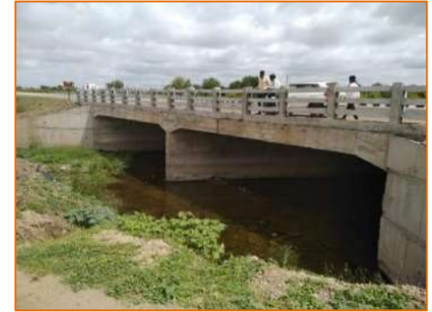
New Minor Bridge at km. 295.622
