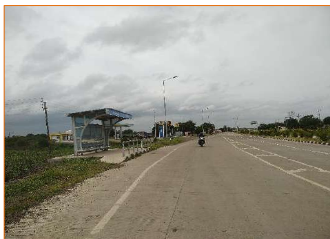
Bus Bay at km. 312+150 (Andhalgaon)
