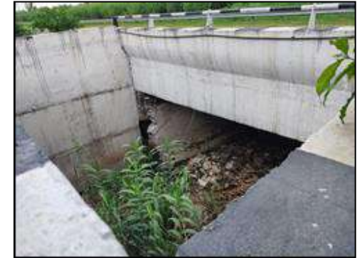
Minor Bridge at km. 76+815 (Structure View)
