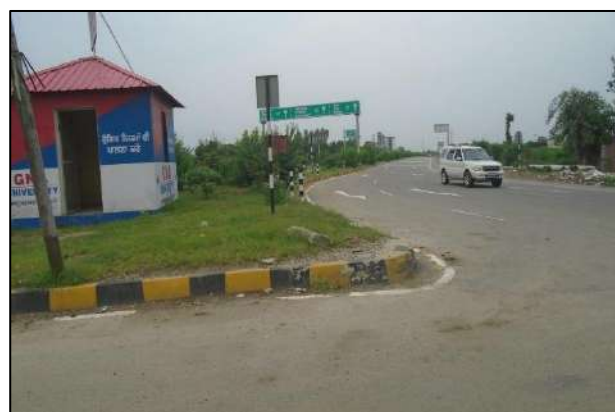
Start of Project Road - Right Carriageway
