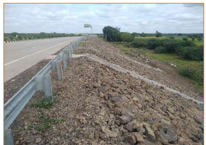
Slope Protection work at km. 298+300
