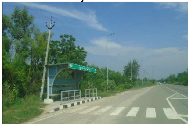
Bus Bay at km. 62+900
