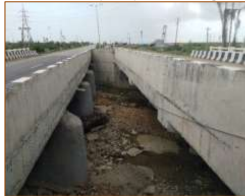
Mid Portion of Minor Bridge at km. 462+447 (LHS) - Widening
