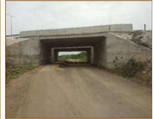
LVUP at km. 488+981 (LHS) - Under COS
