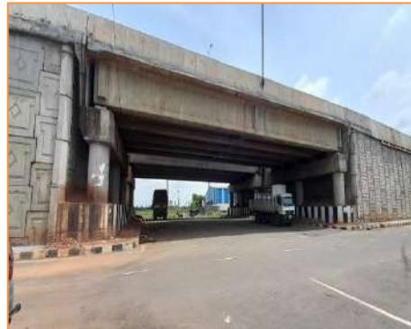
View of VUP at km 83+405
