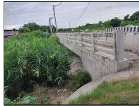
Minor Bridge at km. 75+009 (Structure View)
