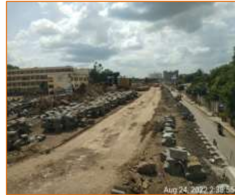
Filling work & RE Block erection work of Flyover is in progress at km. 136.857 @ Akkalkot side (RHS)
