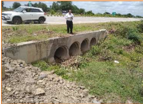
Pipe Culvert at km. 276+190
