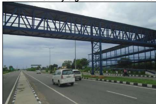
Foot Over Bridge (FOB) at km. 6+600
