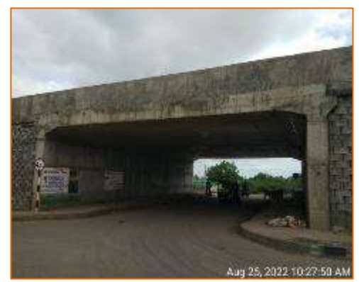
Side View of LVUP at km. 135.100 (RHS)
