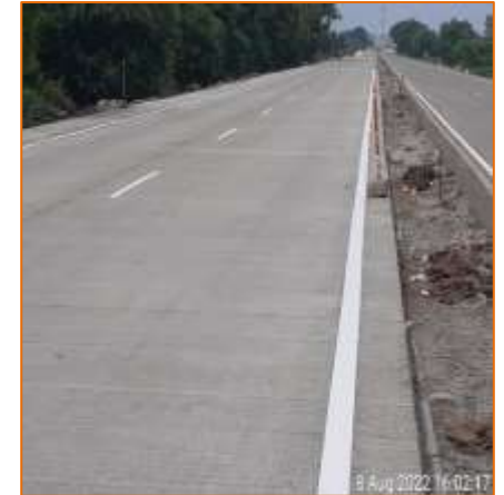
km. 32+450 Work in Progress
