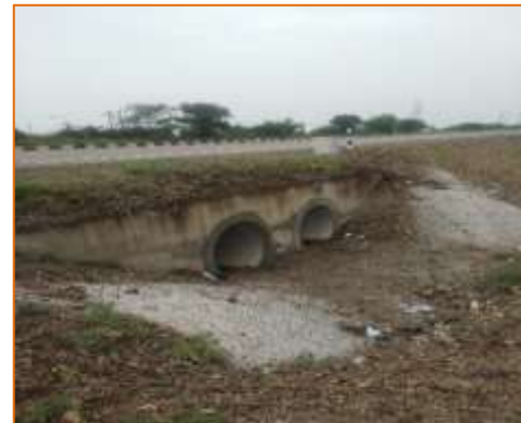
HPC at km. 70+640 (RHS)
