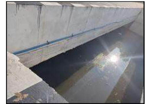
Minor Bridge at km. 71+727 (Structure View)
