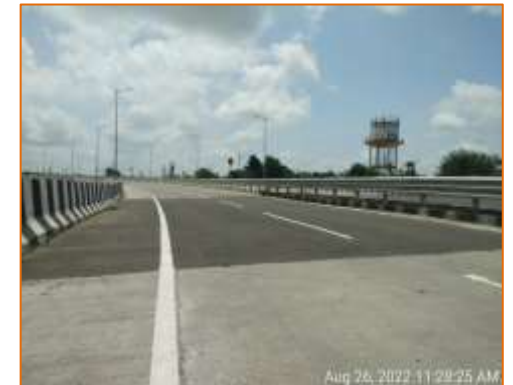
LVUP at km. 114.080 (RHS)
