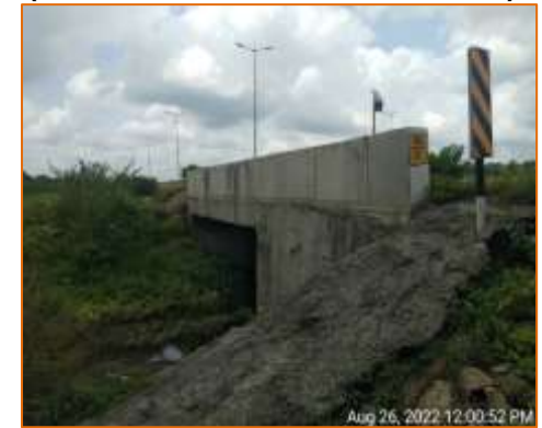
Box culvert at km. 105.290 - LHS (New Construction)
