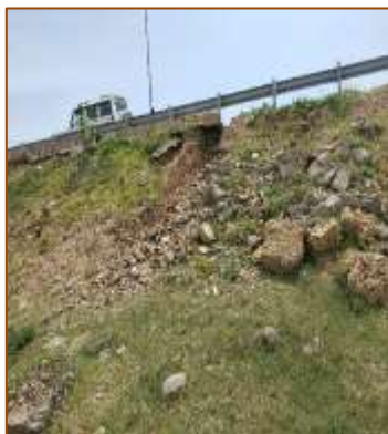
MJB at km. 415+929 (RHS)
