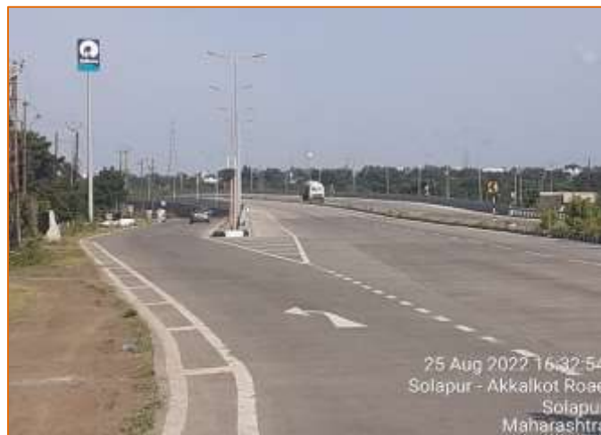
End of the Bypass at km. 106.526
