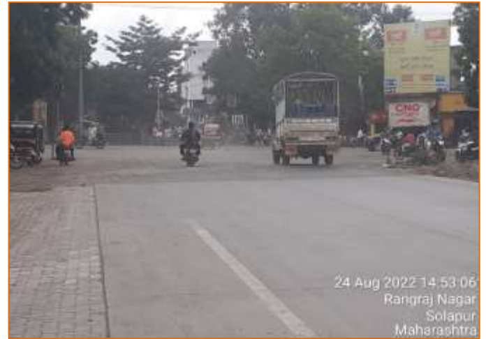
End of the Project Highway at km. 138+352
