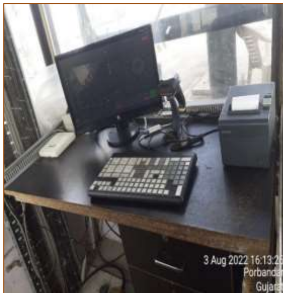
TP-1 at km. 409+500
