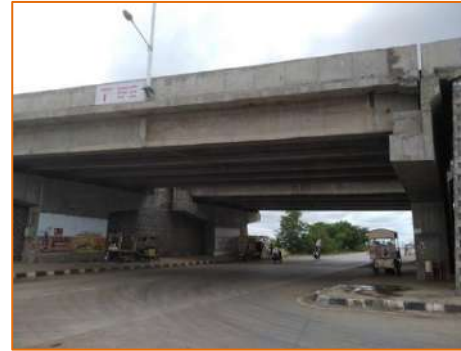
Vehicular Underpass at km. 294.456
