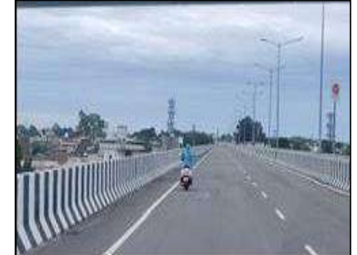
Elevated Structure at km. 25+319
