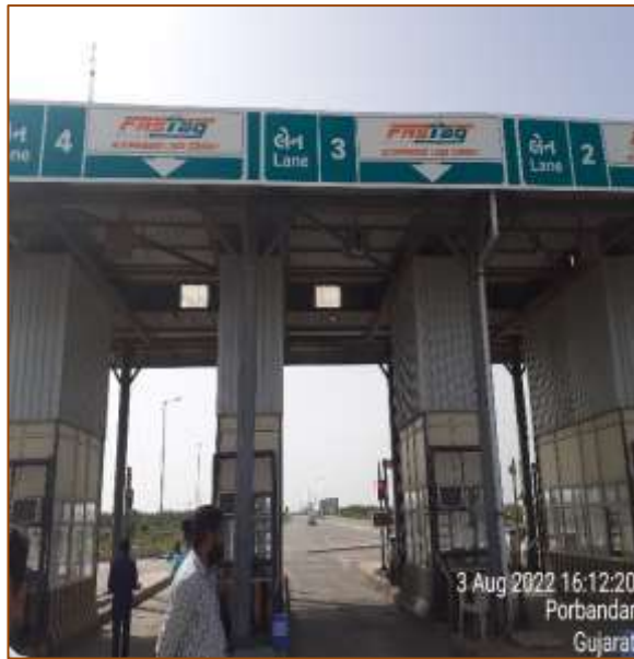
TP-1 at km. 409+500
