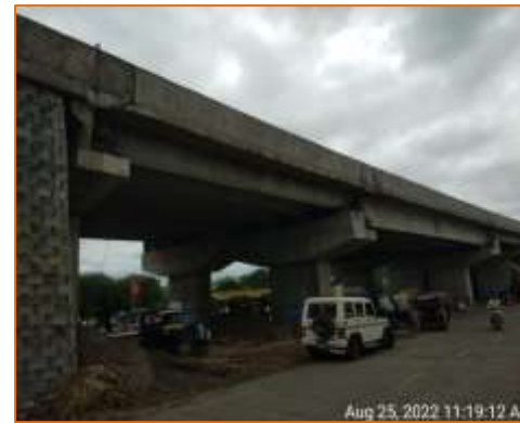
Side View of Flyover at km. 130.650 (LHS)
