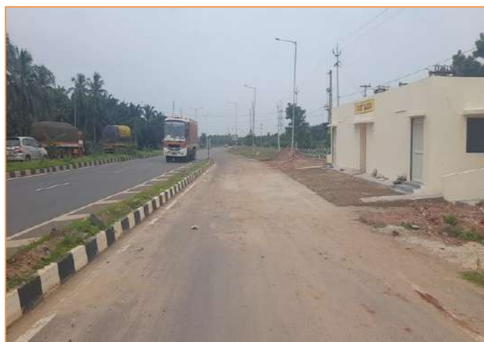
Truck Lay bye at km. 41+500
