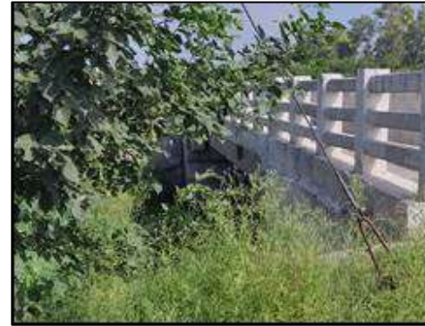
Minor Bridge at km. 63+615 (Existing Structure View)
