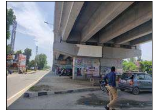
Flyover at km. 59+818
