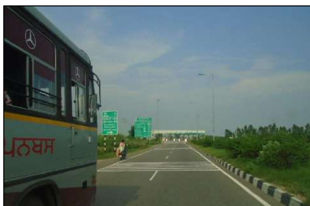
Behram Toll Plaza at km. 15+300
