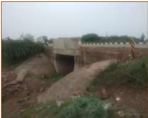
Slab culvert at km. 444+062 (LHS)
