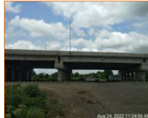
Side View of Flyover at km. 102.700 (RHS)
