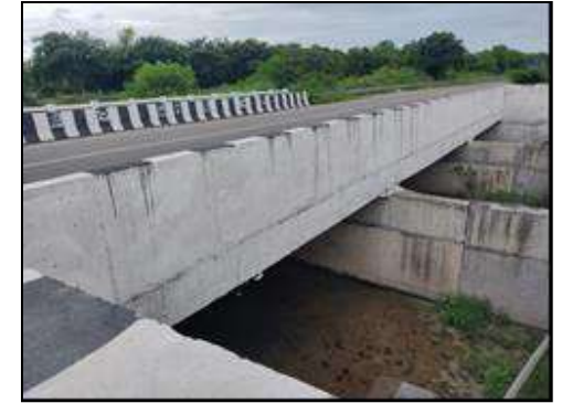
Minor Bridge at km. 72+900 (Top View)
