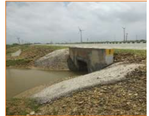
Box culvert at km. 7+240 (RHS)
