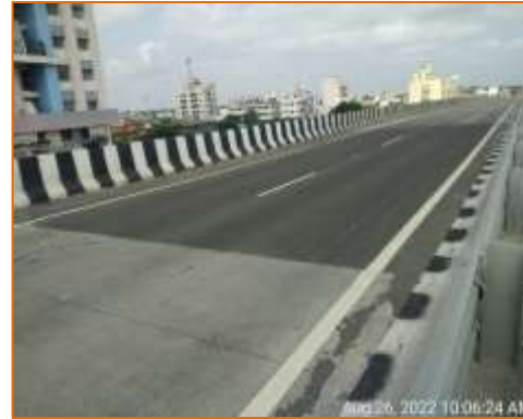
Good BC surface of LVUP at km. 135.100 (LHS)
