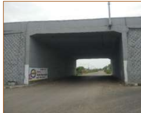
VUP at km. 396+865 (RHS)
