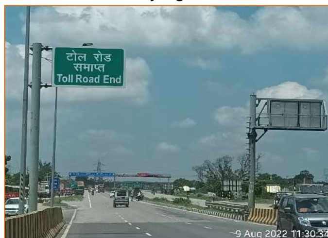
Cantilever Gantry Sign at km. 713+000.
