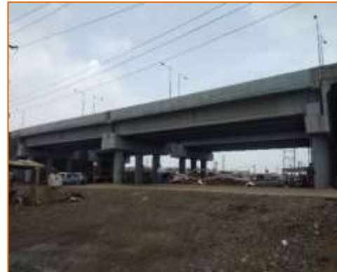
Side View of VUP at km. 12+420 (LHS)
