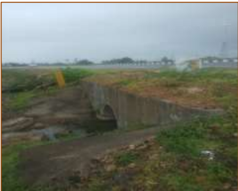
HPC at km. 437+025 (LHS)
