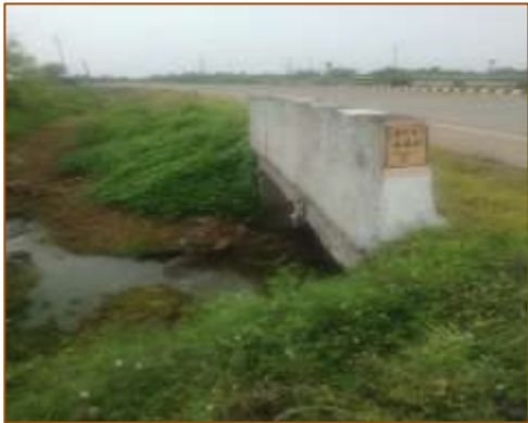
Slab culvert at km. 439+458 (LHS)
