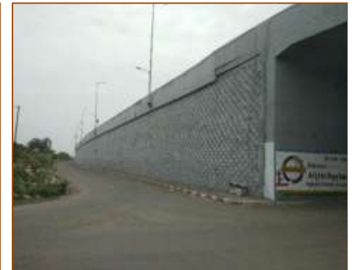
VUP at km. 396+865 (RHS) - A1 side
