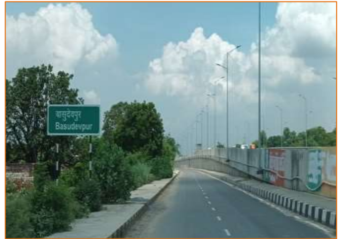
Drain at Service Road at km. 757+200
