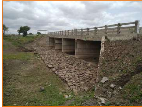
New Minor Bridge at km. 282.548
