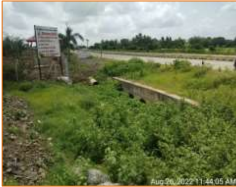
Pipe Culvert at km. 109.578 - RHS (Widening)
