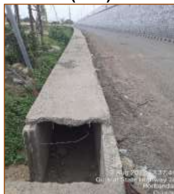
Built-up drain from km. 400+319 to 400+700 (LHS)
