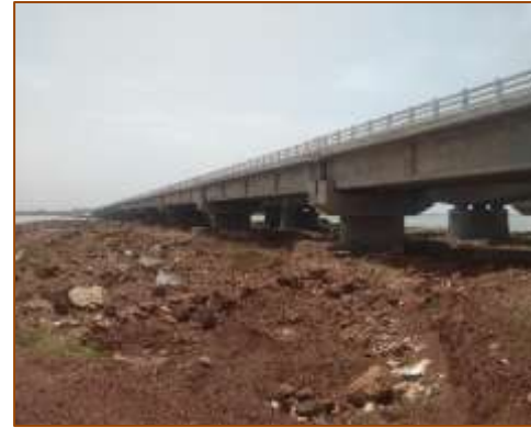
Major Bridge - km. 433+295 (RHS) side view
