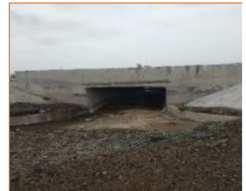
Box culvert at km. 62+720 (RHS)
