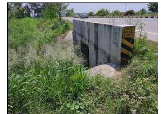
Box Culvert at km. 53+510
