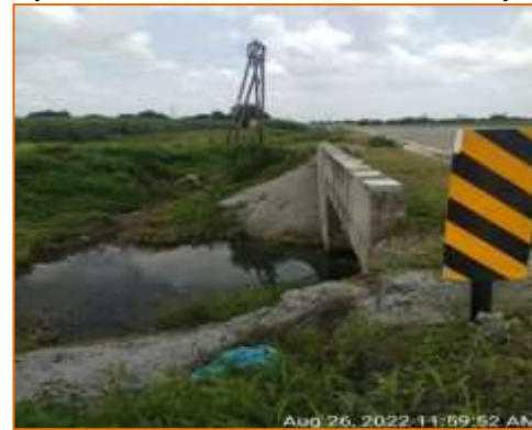
Box culvert at km. 105.290 - RHS (New Construction)
