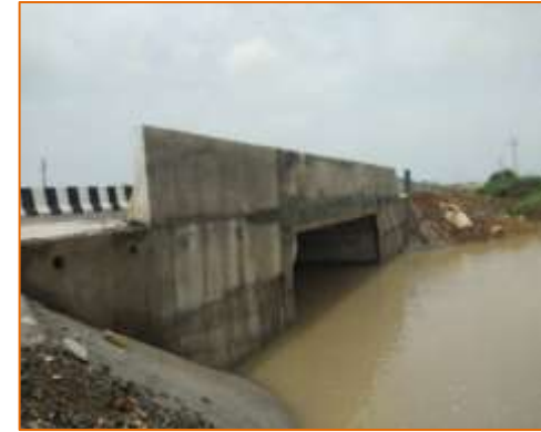
Side View of Minor Bridge at km. 9+880 (LHS)
