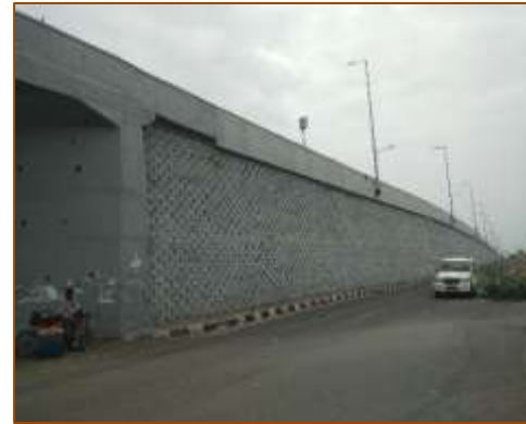
VUP at km. 397+096 (LHS) - Skew - A1 side
