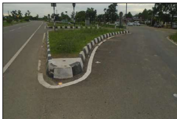
Major Junction at km. 57+260 (RHS)
