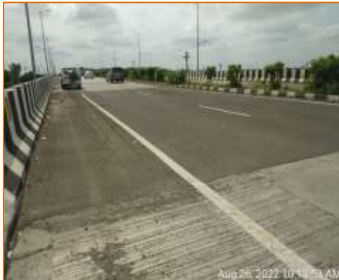
LVUP at km. 132.025 (RHS)
