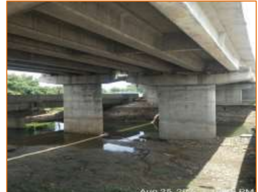
Bottom of Minor Bridge at km. 117.796 - BHS (MCW)
