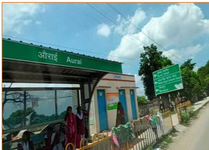
Toilet Block at km. 754+130
