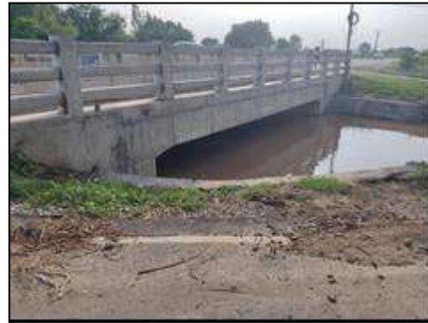
Minor Bridge at km. 35+812 (New Structure View)
