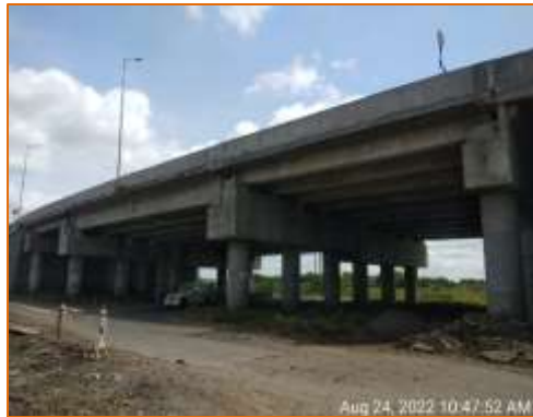
Side View of Flyover at km. 99.900 (LHS)
