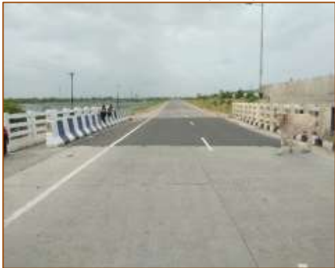
Minor Bridge at km. 406+170 (RHS) - Widening - Wearing Coat
