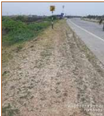
From km. 408+000 to km. 409+000 (RHS)
