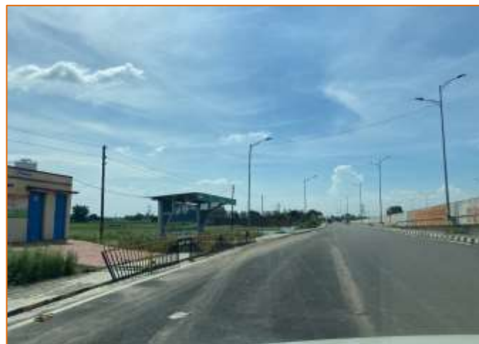
Toilet Block at km. 775+910
