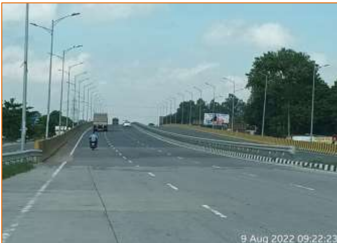
Highway Lighting at km. 773+100
