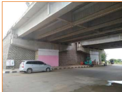
Vehicular Underpass at km. 292.230
