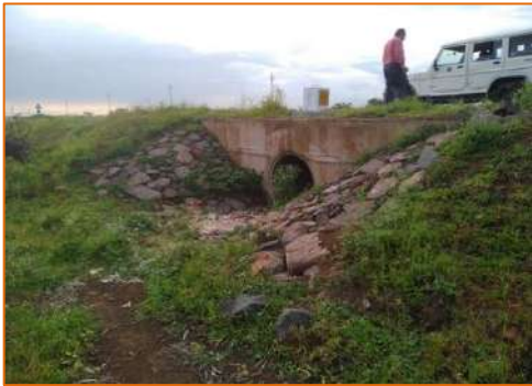
Pipe Culvert at km. 300+020
