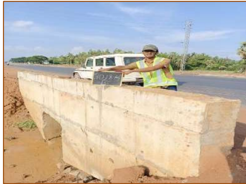
Box Culvert at km. 30+874
