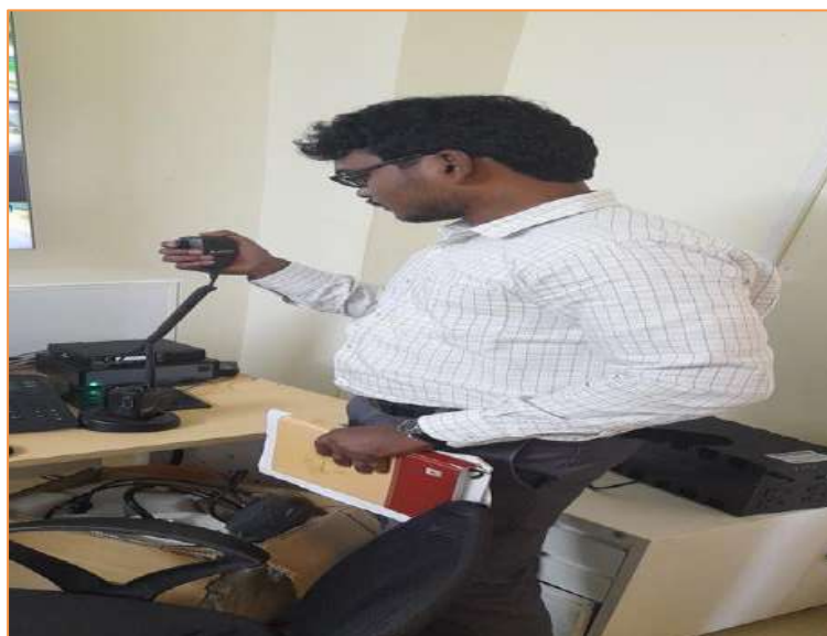
Figure 3-19 Emergency communication system is checking at Toll plaza
