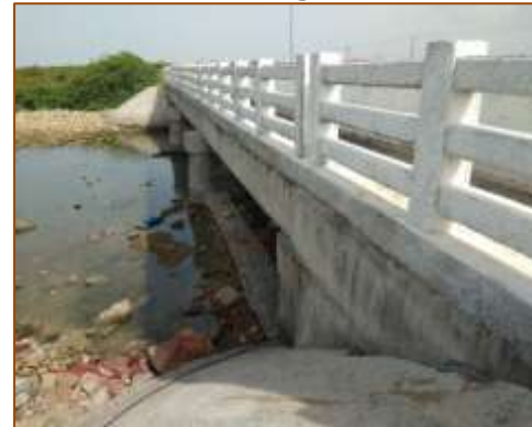
Side View of Minor Bridge at km. 494+166 (LHS) - Widening
