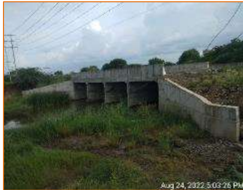
Side View of MNB at km. 99.586 (RHS)
