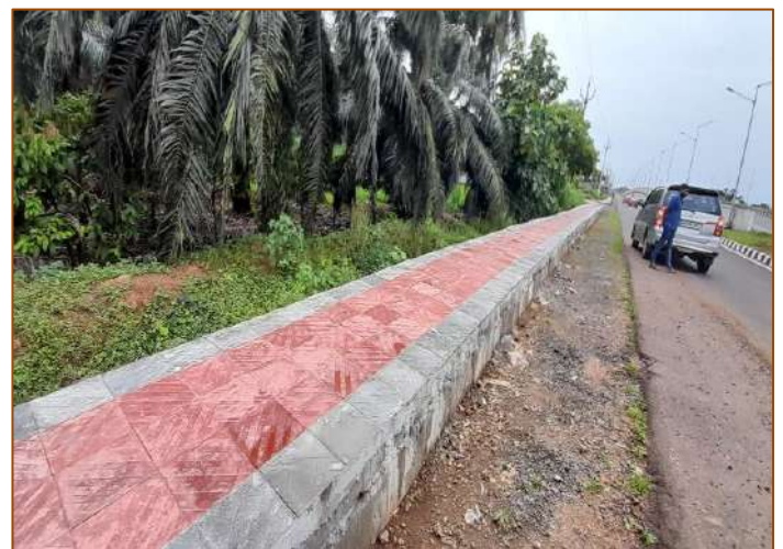
Built-up Drain cum footpath at km. 36+450
