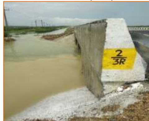
Side View of Minor Bridge at km. 1+620 (RHS)
