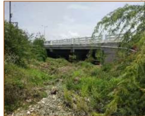
Side View of Minor Bridge at km. 440+350 (LHS) - New
