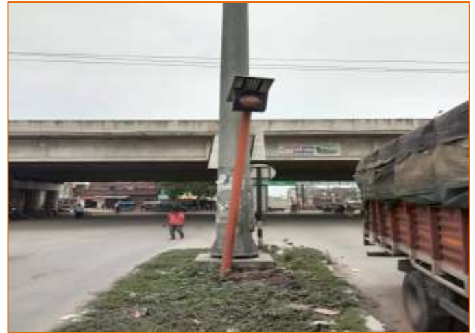
LED Blinker at km. 754+441
