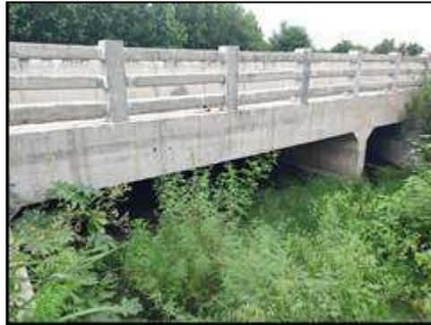
Minor Bridge at km. 74+361 (Structure View)
