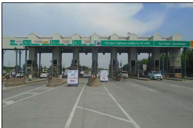
Bachhwan Toll Plaza at km. 70+240
