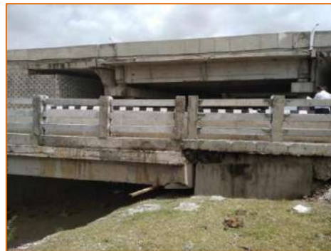
New Minor Bridge at km. 292.148
