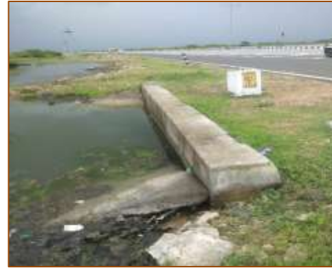
HPC at km. 391+096 (LHS)
