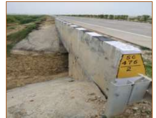
Slab culvert at km. 475+860 (RHS)
