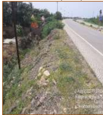
From km. 443+000 to km. 444+000 (RHS)
