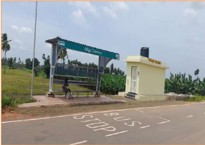
Bus Bay with Shelter at km. 79+200
