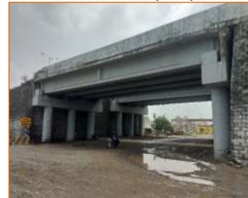
Side View of VUP at km. 57+975 (LHS)
