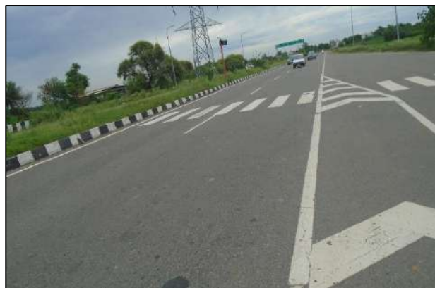
Road Marking at km. 15+800 (RHS)
