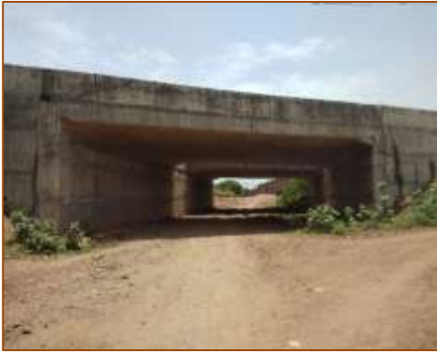
LVUP at km. 381+600 (RHS) - Under COS
