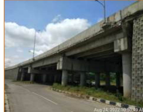
Side View of Flyover at km. 99.900 (RHS)
