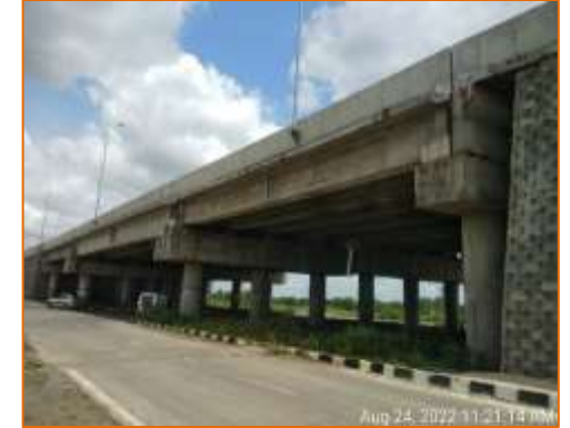
Side View of Flyover at km. 102.700 (LHS)
