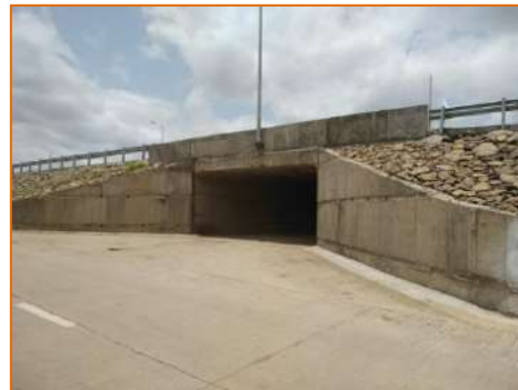
Pedestrian Underpass at km. 284.500
