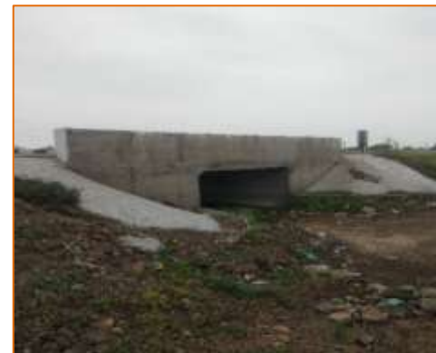
Box culvert at km. 62+720 (LHS)
