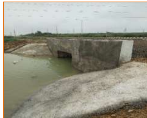
Box culvert at km. 11+950 (RHS)
