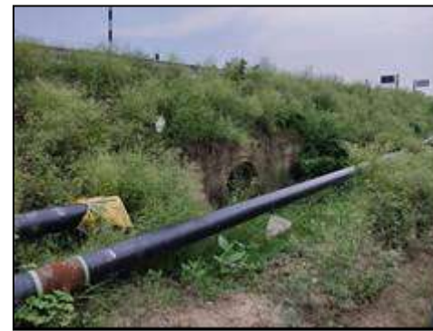
HP Culvert at km. 1+135
