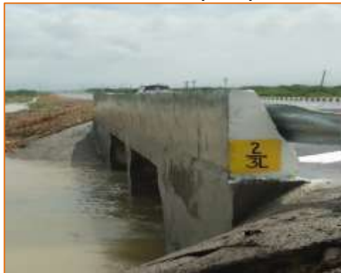
Side View of Minor Bridge at km. 1+620 (LHS)
