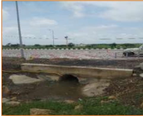
HPC at km. 5+800 (RHS)
