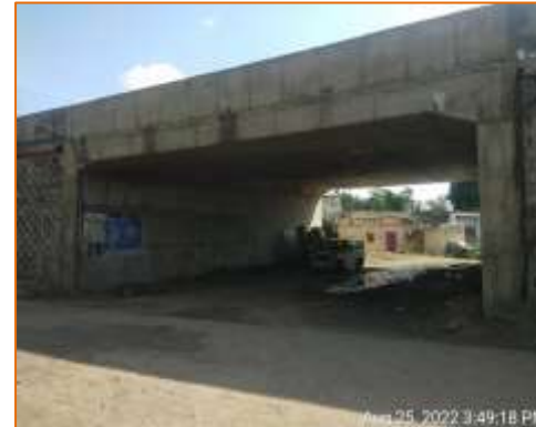
Side view of LVUP at km. 114.080 (RHS)
