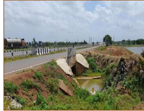
Box Culvert at km. 35+736
