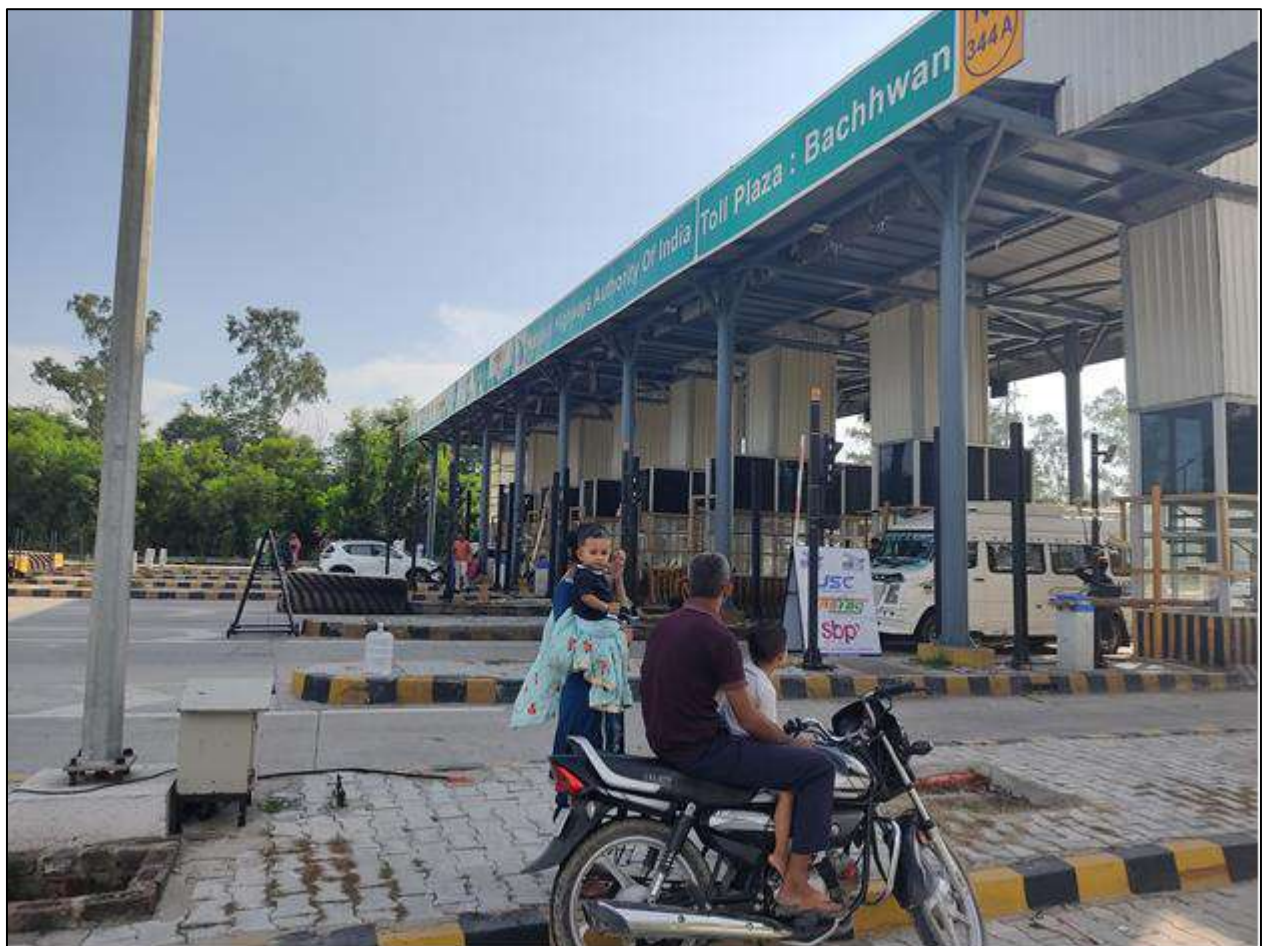
Figure 9-2 View of Bachhwan Toll Plaza (km. 70+240)
