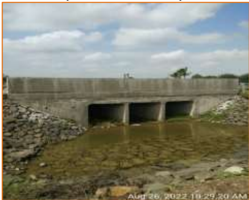
Box culvert at km. 128.229 - RHS (Reconstruction)
