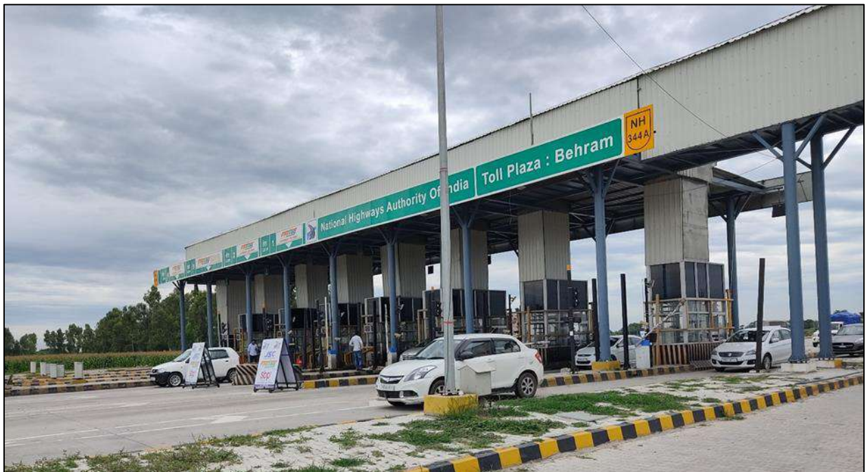
Figure 9-1 View of Behram Toll Plaza (km. 15+300)
