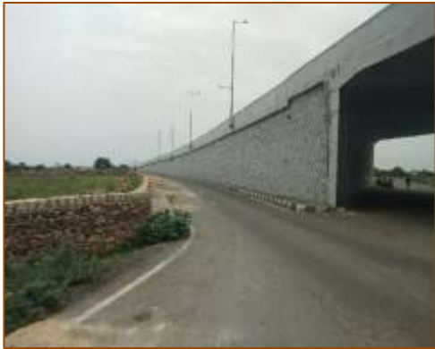
VUP at km. 397+096 (RHS) - Skew - A1 side
