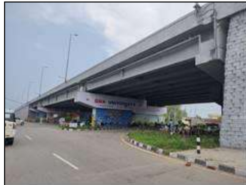
Flyover at km. 4+225
