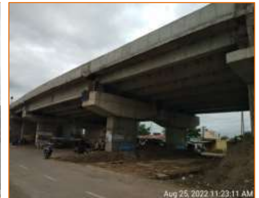
Side View of Flyover at km. 130.650 (RHS)
