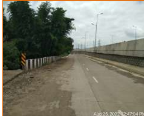
Good condition of PQC surface of MNB at km. 121.678 - LHS (SR)
