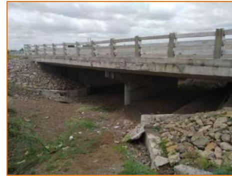
New Minor Bridge at km. 289.260
