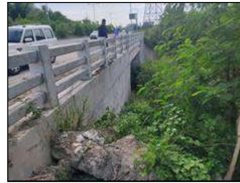
Minor Bridge at km. 69+815 (New Structure View)
