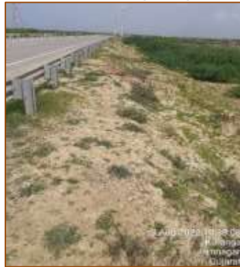
From km. 466+000 to km. 467+000 (RHS)
