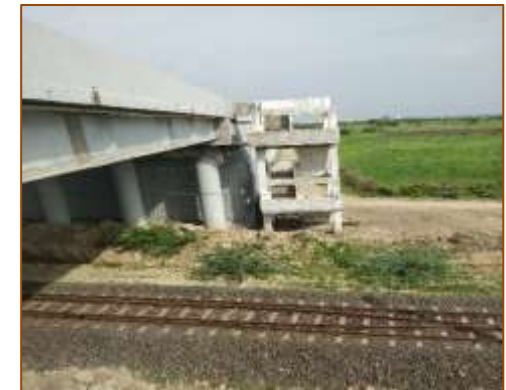
Side View of ROB at km. 393.642 (LHS)
