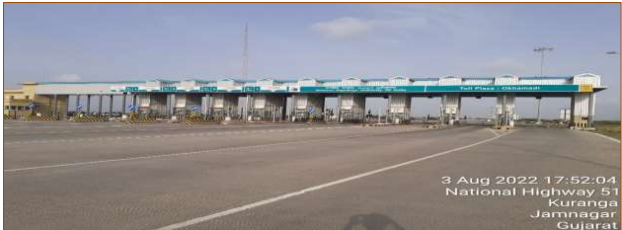
Figure 9-2 View of Okhamadi Toll Plaza
