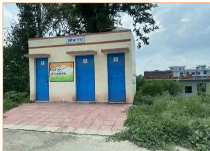
Toilet Block at km. 768+420
