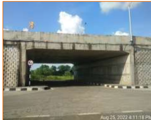
Side view of LVUP at km. 111.260 (LHS)
