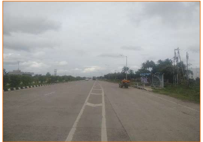
Bus Bay at km. 301+600 (Dighewadi)
