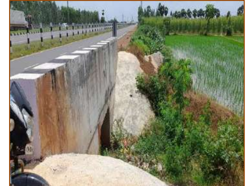
Box Culvert at km. 56+650
