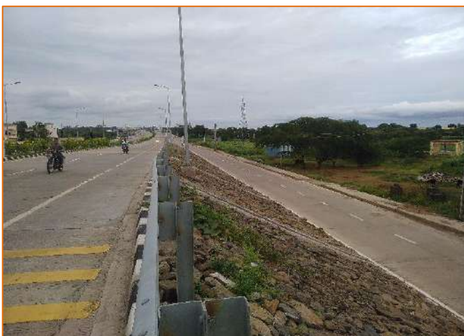
Slope Protection work at km. 284+500.000
