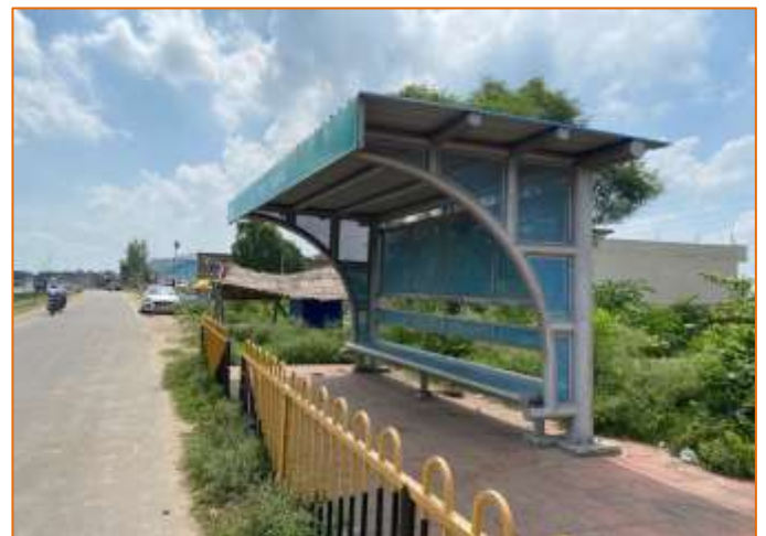
Bus Shelter at km. 767+915
