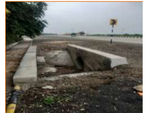
HPC at km. 70+640 (LHS)
