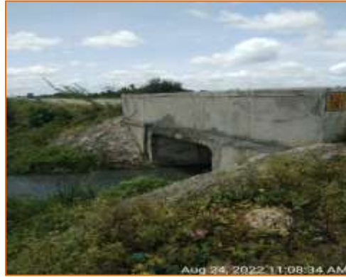
Box culvert at km. 101.823 - RHS (New Construction)
