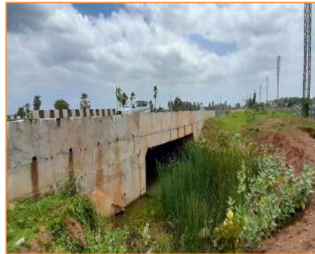
View of Minor Bridge at km. 26+850
