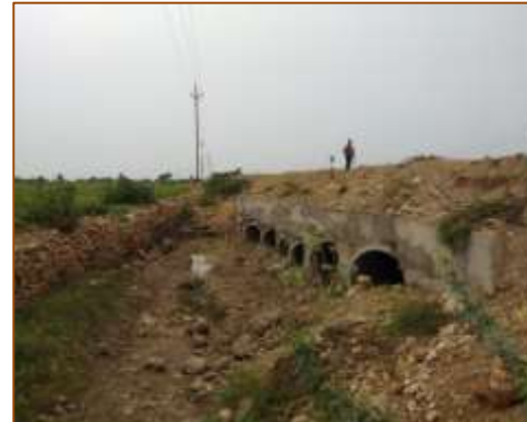
HPC at km. 456+200 (LHS)
