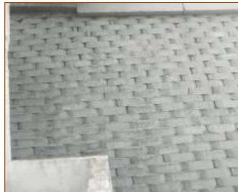
Vertical crack developed at A2 side at km. 393+642 - ROB (RHS)
