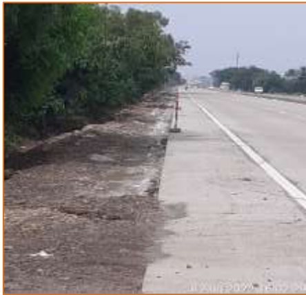
km. 32+450 Work in Progress
