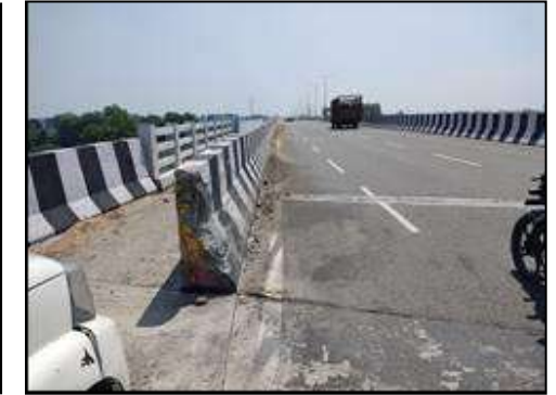
Minor Bridge at km. 38+326 (New Structure 4-lane View)
