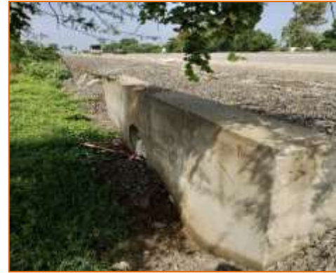
HPC at km. 32+520 (RHS)
