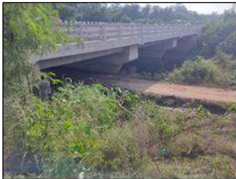
Minor Bridge at km. 71+174 ( Structure View)
