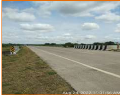
PQC of Minor Bridge at km. 101.260 (LHS)
