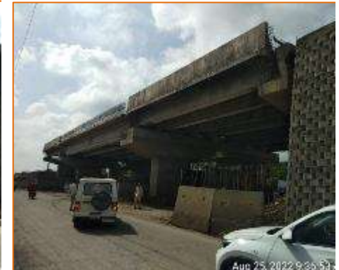
Side View of Flyover at km. 136.857 (RHS)
