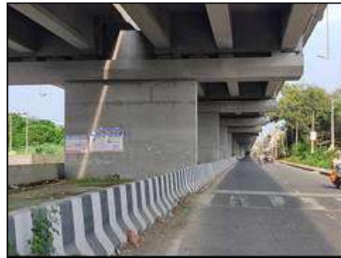
Elevated Structure at km. 25+319
