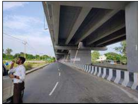
Elevated Structure at km. 25+319
