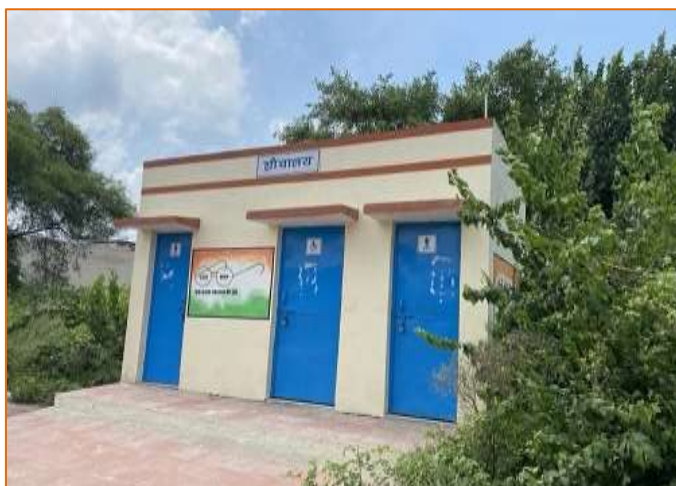
Toilet Block at km. 764+770
