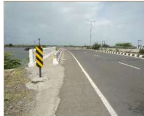
Minor Bridge at km. 406+880 (RHS) - Widening - Wearing Coat
