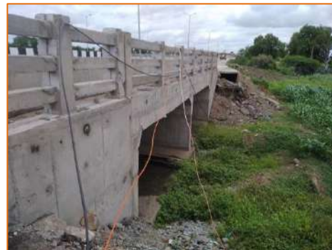
Reconstruction of Minor Bridge at km. 284.835
