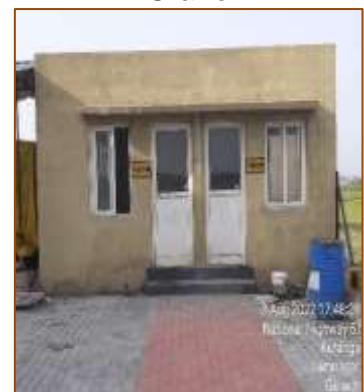
Panel / Pump Room
