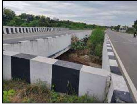
Minor Bridge at km. 72+134 (Top View)
