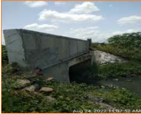
Box culvert at km. 101.823 - LHS (New Construction)
