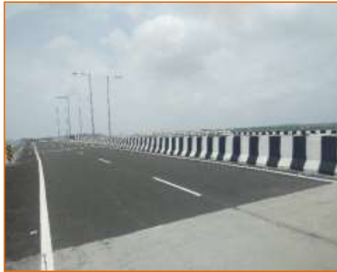
Wearing Coat of ROB at km. 0+527 (RHS)
