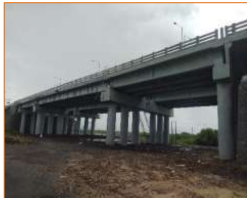
Side View of ROB at km. 0+527 (LHS)
