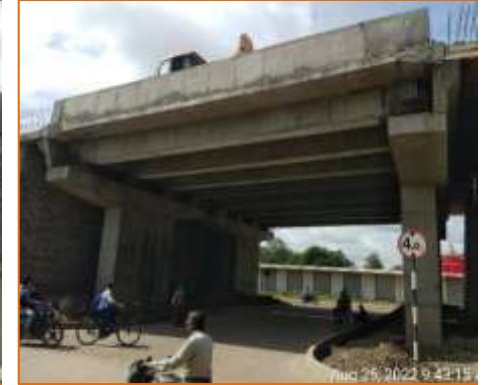
Side View of PUP at km. 136.657 (RHS)
