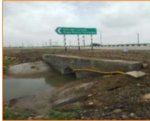
HPC at km. 5+800 (LHS)
