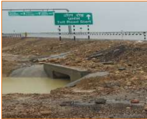
Box culvert at km. 0+060 (LHS)
