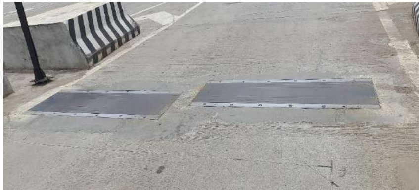
Figure 9-11 Medium Speed Weigh in Motion (MSWIM)
