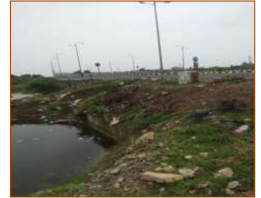
HPC at km. 391+096 (RHS)
