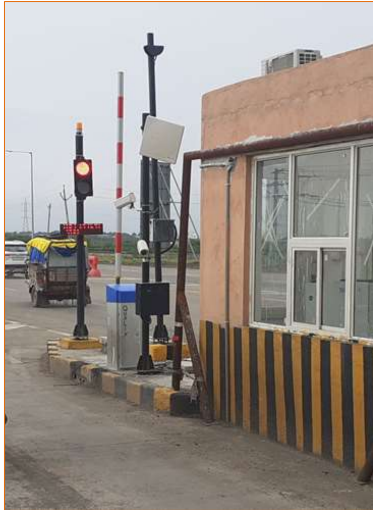
Figure 8-2 RFID Scanner located on pole
