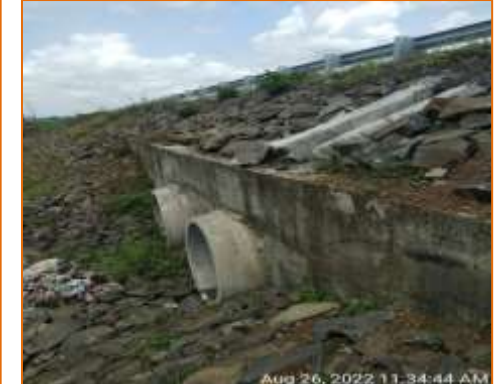
Pipe Culvert at km. 113.155-LHS (Widening)
