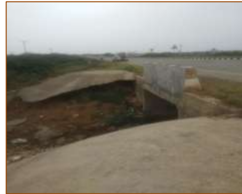
Slab culvert at km. 441+648 (LHS)
