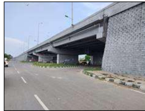
Flyover at km. 9+335
