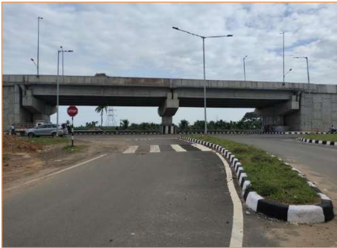
Highway Lighting at km. 45+645
