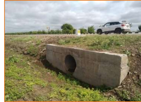
Pipe Culvert at km. 292+135
