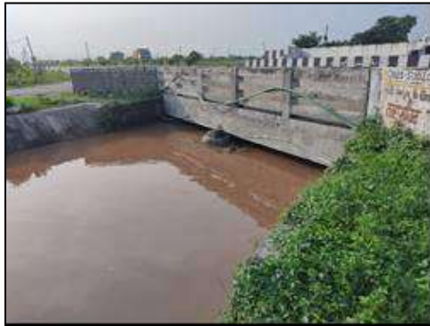
Minor Bridge at km. 35+812 (Existing Structure View)
