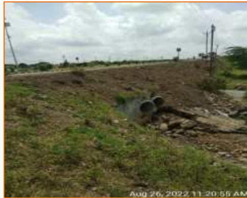
Pipe Culvert at km. 117.423 - LHS (Widening)
