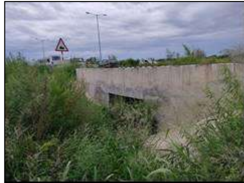
Box Culvert at km. 36+929
