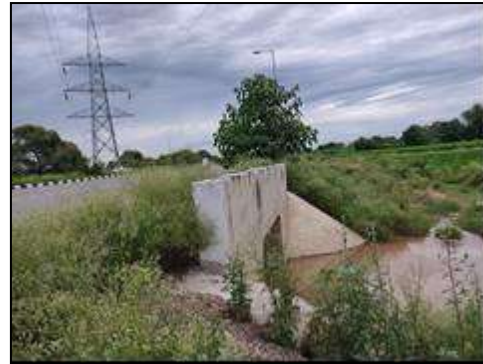
Box Culvert at km. 17+946
