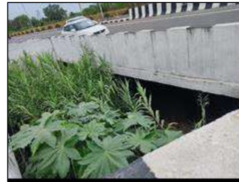
Minor Bridge at km. 78+636 (Structure View)
