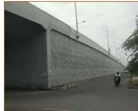
VUP at km. 400+681 (LHS) at A1 side
