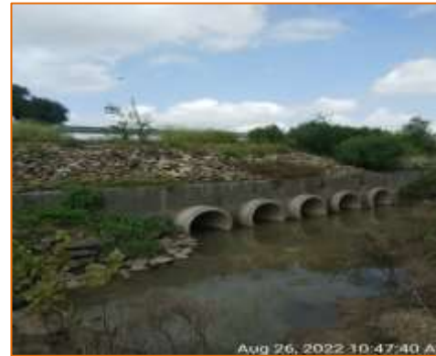
Pipe Culvert at km. 124.106 - RHS (Widening)
