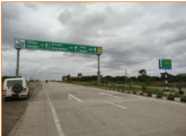
End of Project Road at km. 321.600
