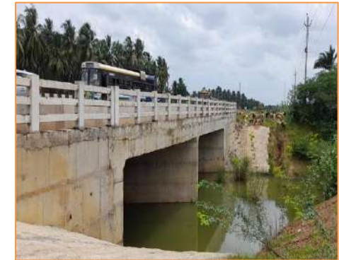
View of Minor Bridge at km. 30+774
