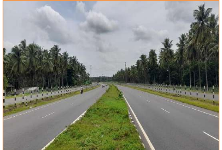
Pavement Condition at km. 46+700
