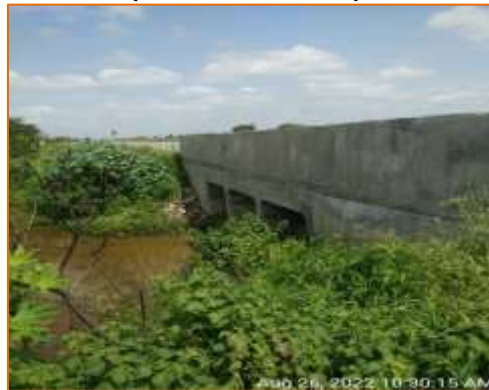
Box culvert at km. 128.229 - LHS (Reconstruction)
