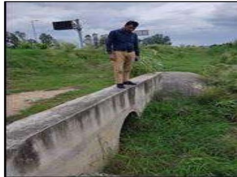
HP Culvert at km. 69+420
