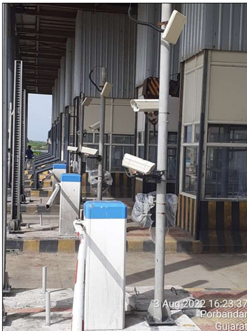
Figure 9-3 RFID ETC Reader mounted on Pole
