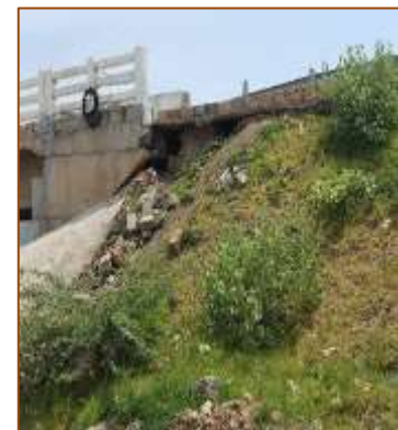
MJB at km. 415+929 (RHS)
