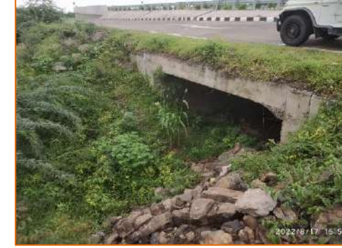
Box Culvert at km. 311.734
