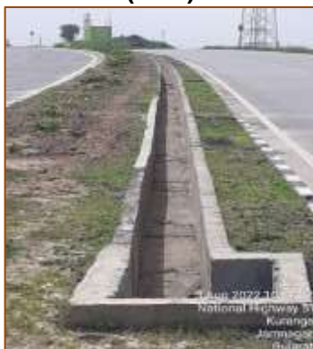
Median longitudinal drain from km. 472+000 to km. 473+000
