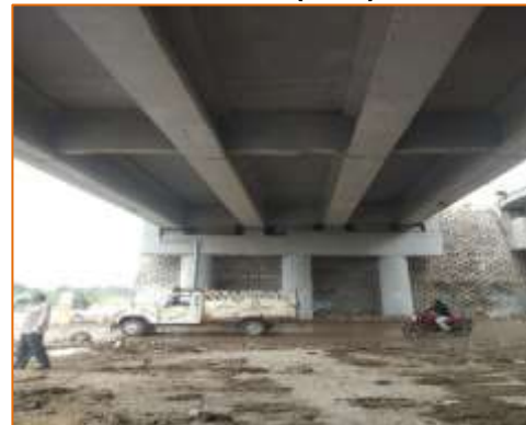
Bottom View of VUP at km. 55+300
