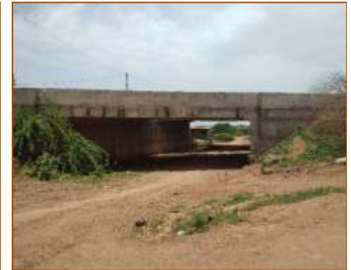
LVUP at km. 488+981 (RHS) - Under COS
