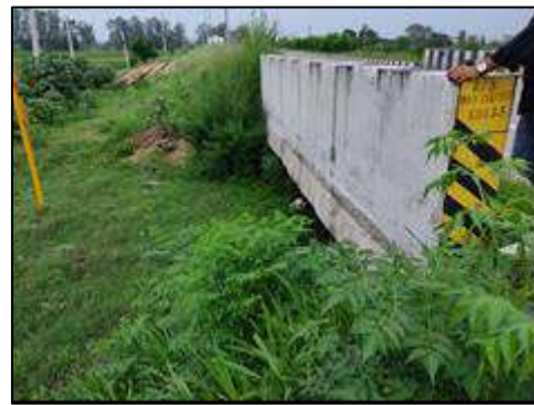
Box Culvert at km. 1+457
