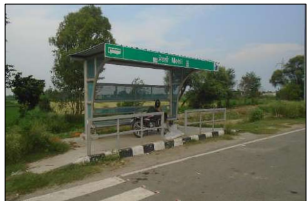
Bus Bay at km. 10+255
