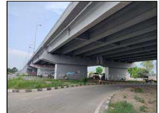
Flyover at km. 9+335
