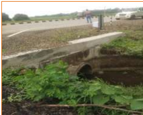
HPC at km. 66+010 (RHS)
