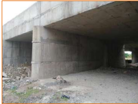
Widening of Existing Minor Bridge at km. 281.277
