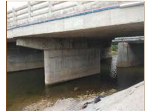
Bottom of Minor Bridge at km. 455+195 (RHS)
