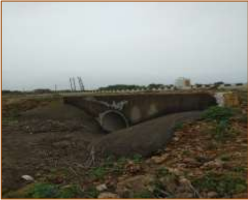
HPC at km. 380+328 (LHS)
