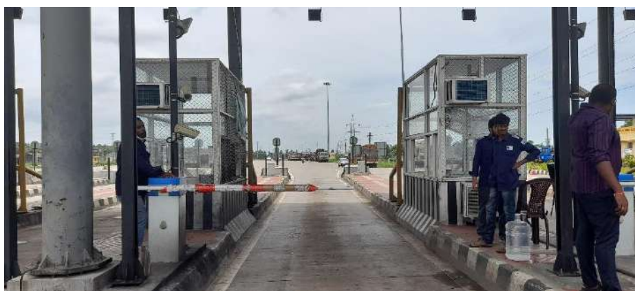
Figure 9-6 Automatic Lane Barrier
