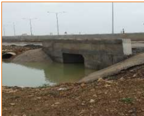
Box culvert at km. 11+950 (LHS)
