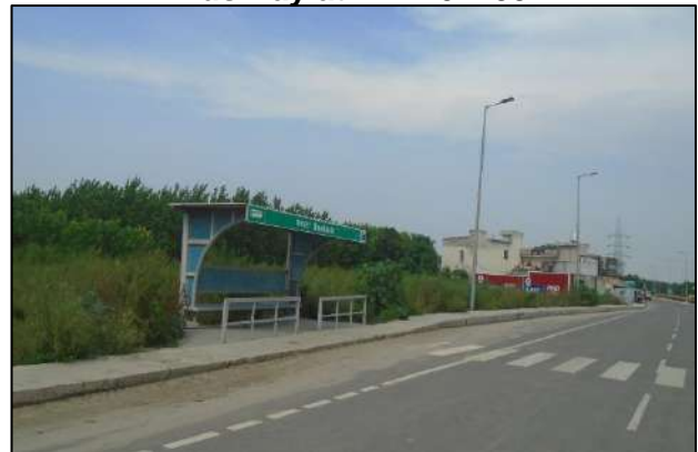
Bus Bay at km.69+200
