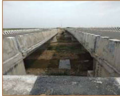
Mid Portion of Major Bridge at km. 395+255
