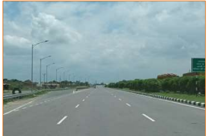
Truck Lay Bye at km. 767+330
