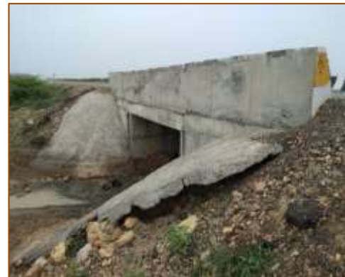
Slab culvert at km. 475+860 (LHS)
