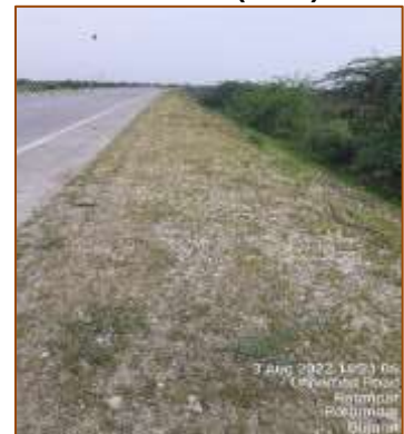
From km. 384+000 to km. 385+000 (RHS)
