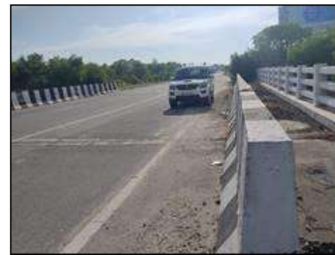
Minor Bridge at km. 71+727 (Top View)
