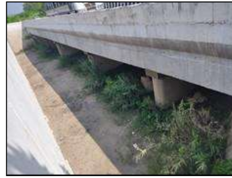
Minor Bridge at km. 64+791 (Existing Structure View)
