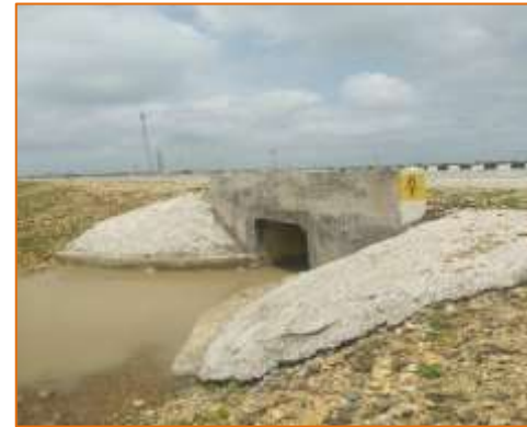
Box culvert at km. 7+240 (LHS)
