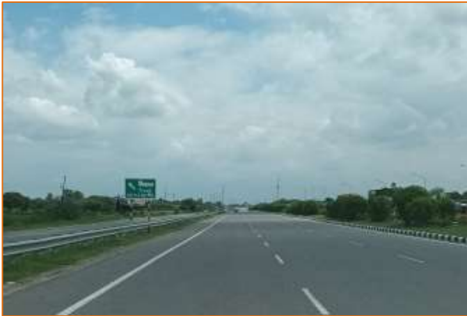
Truck Lay Bye at km. 727+900
