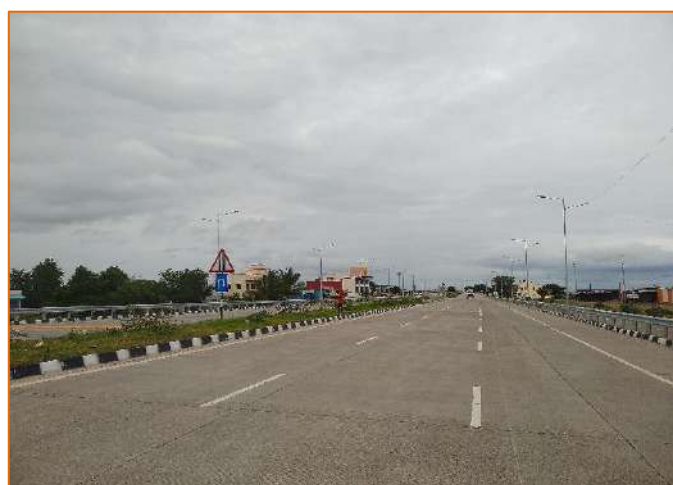
Road Markings at km. 286+600
