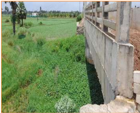
View of Minor Bridge at km. 24+603
