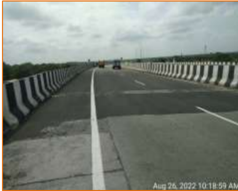
Good condition of BC surface of Flyover at km. 130.650 (RHS)
