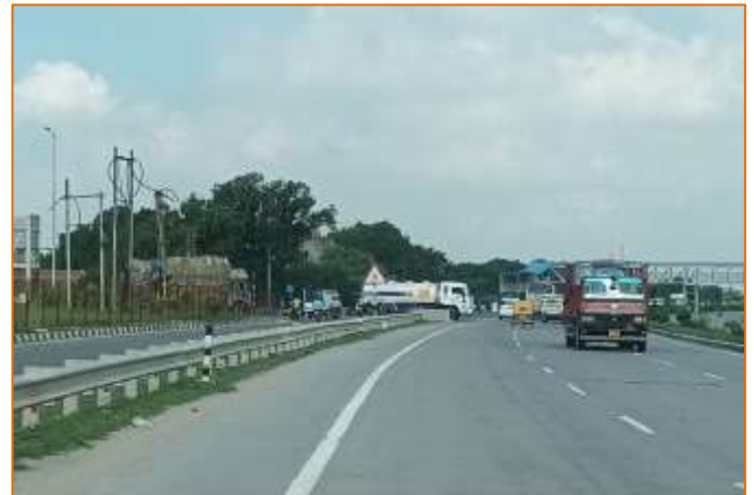
Crash Barrier at km. 782+000
