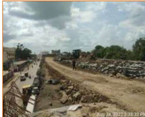
Filling work & RE Block erection work of Flyover is in progress at km. 136.857 @ Akkalkot side (LHS)
