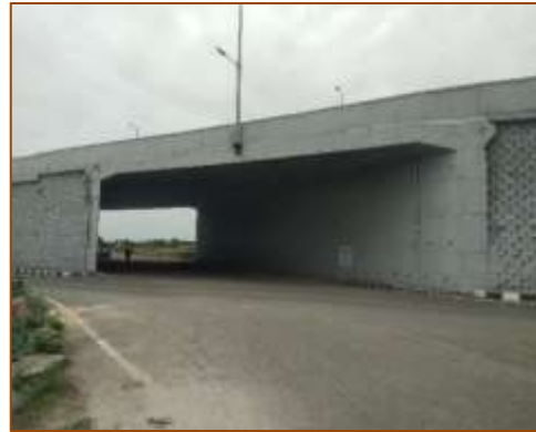
VUP at km. 397+096 (RHS)
