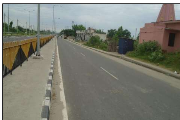
Service Road at km. 77+600 (LHS)
