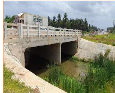
View of Minor Bridge at km. 28+782
