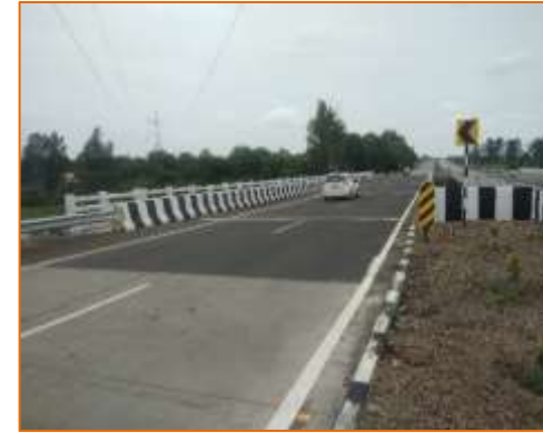
Wearing Coat of Major Bridge at km. 66+310 (RHS)
