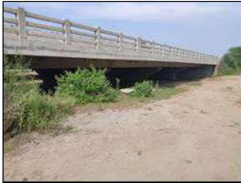
Minor Bridge at km. 68+519 (Existing Structure View)
