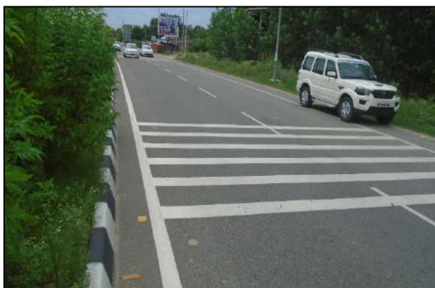
Road Marking at km. 70+000 (RHS)
