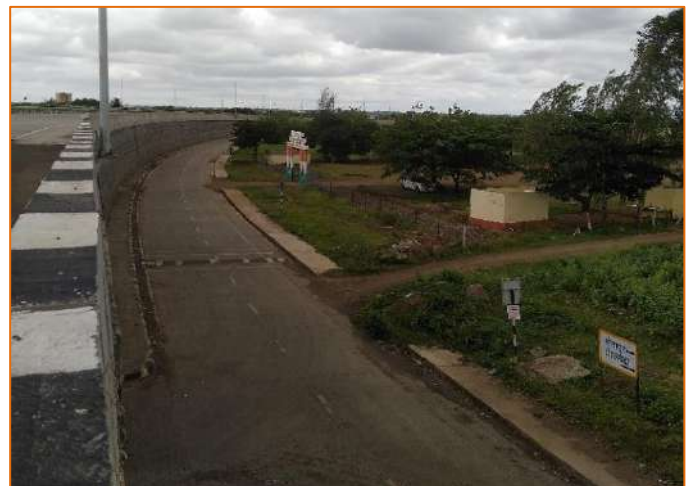
Built-up Drain at km. 299+350
