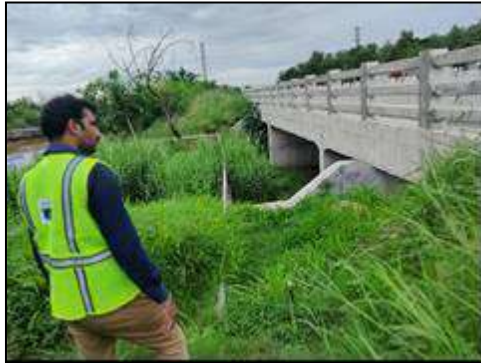
Minor Bridge at km. 74+173 (Structure View)
