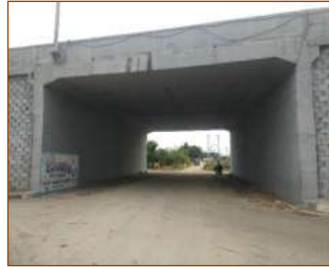
LVUP at km. 422+750 (LHS) - Under COS
