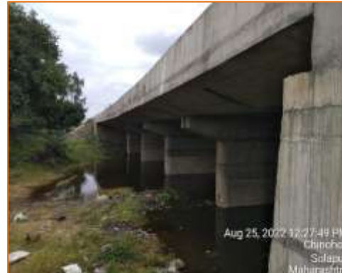
Side View of Minor Bridge at km. 124.337 (RHS)
