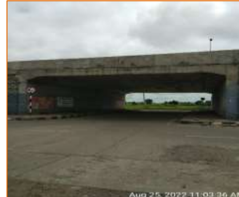
Side View of LVUP at km. 132.025 (LHS)
