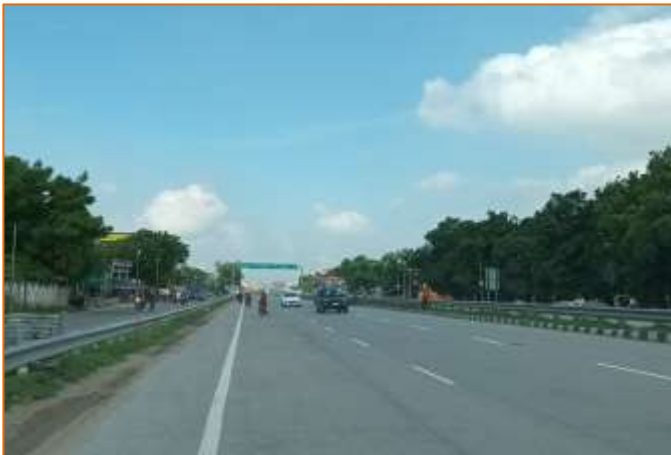
Crash Barrier at km. 785+240
