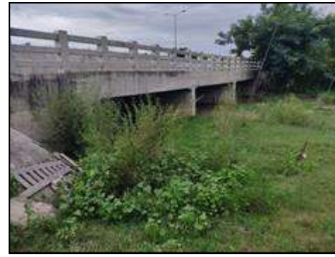
Minor Bridge at km. 72+900 (Structure View)
