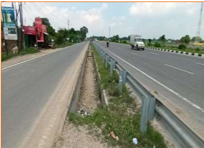
RCC Open Drain at km. 762+000
