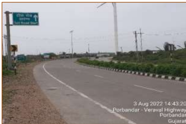
Porbandar Bypass at km. 379.100
