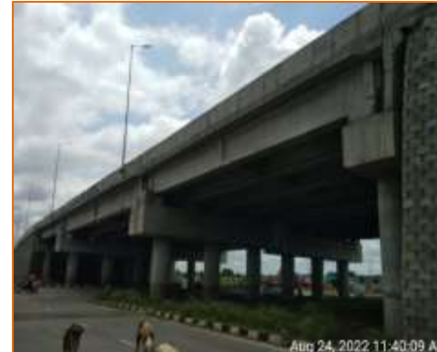
Side View of Flyover at km. 103.801 (RHS)
