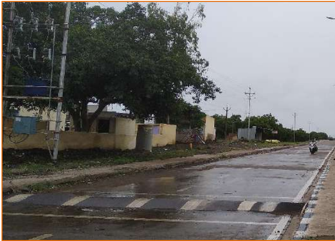
Built-up Drain at km. 314+735
