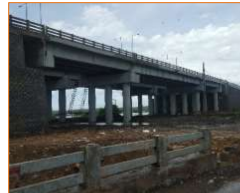
Side View of ROB at km. 0+527 (RHS)
