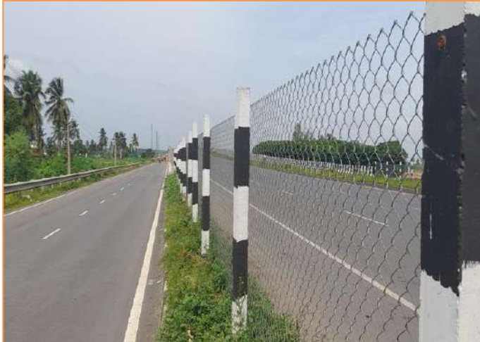
Chain fencing at km. 85+150
