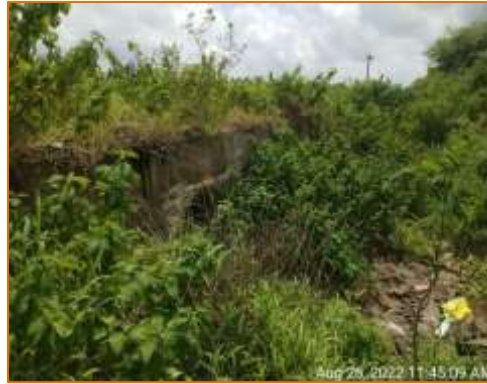
Pipe Culvert at km. 109.578 - LHS (Widening)
