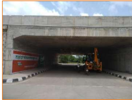
Light Vehicular Underpass at km. 288.116
