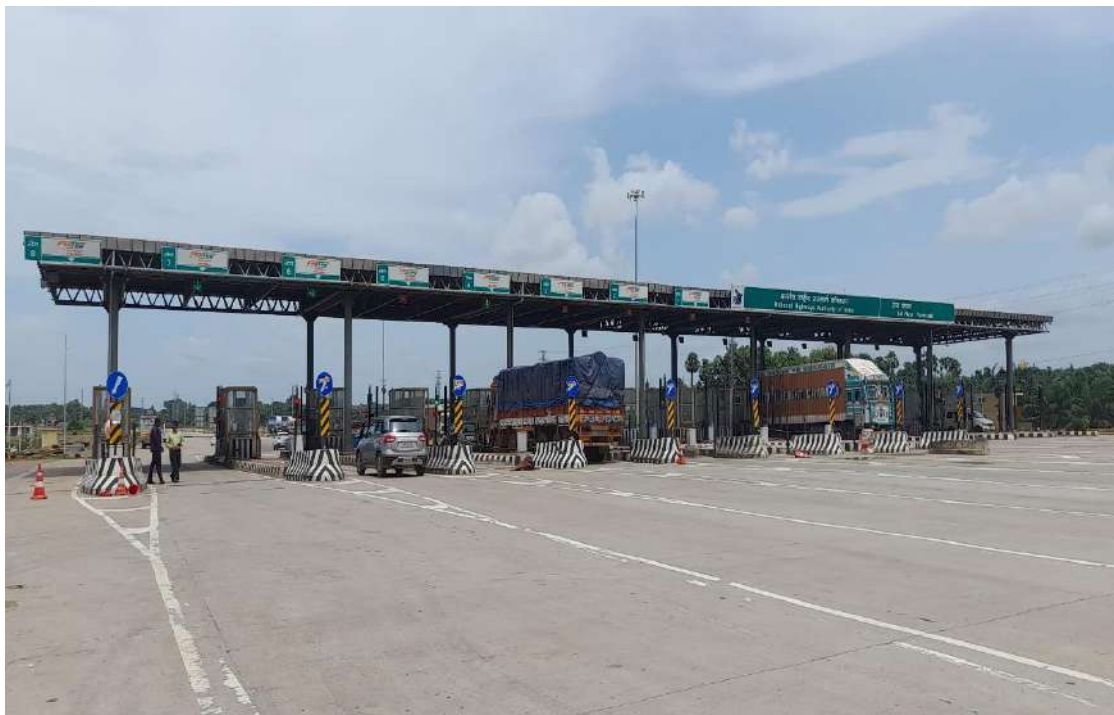
Figure 9-1 View of Toll Plaza (km. 53+700)
