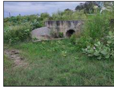
HP Culvert at km. 1+850
