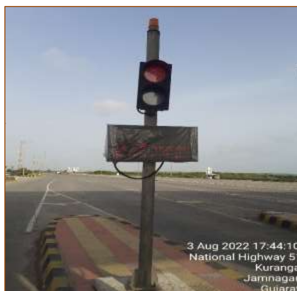
TP-2 at km. 470+875
