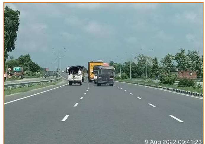
Road Marking at km. 761+200.
