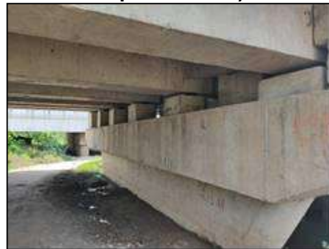
Minor Bridge at km. 71+174 (Substructure and Superstructure)
