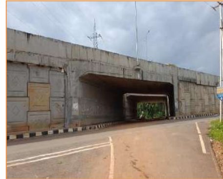
View of LVUP at km 44+135
