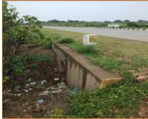
HPC at km. 380+328 (RHS)
