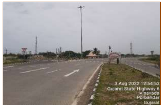
Visawada Bypass at km. 422.800
