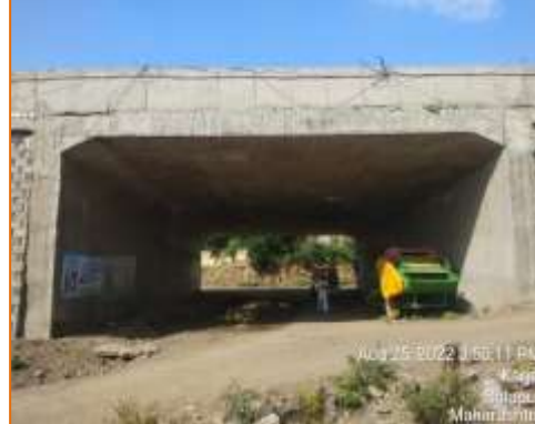
Side view of LVUP at km. 114.080 (LHS)
