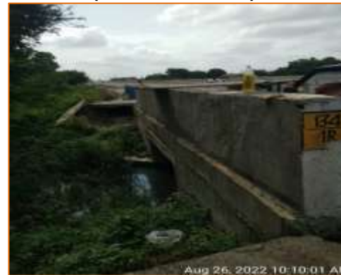
Box culvert at km. 133.524 - RHS (Reconstruction)
