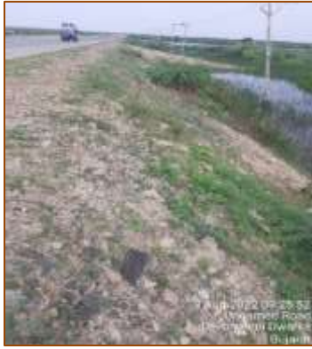
From km. 492+000 to km. 493+000 (RHS)
