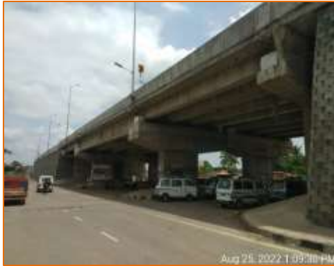
Side View of Flyover at km. 117.935 (LHS)
