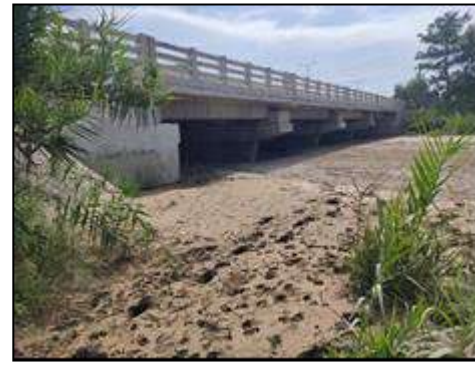
Minor Bridge at km. 68+519 (New Structure View)
