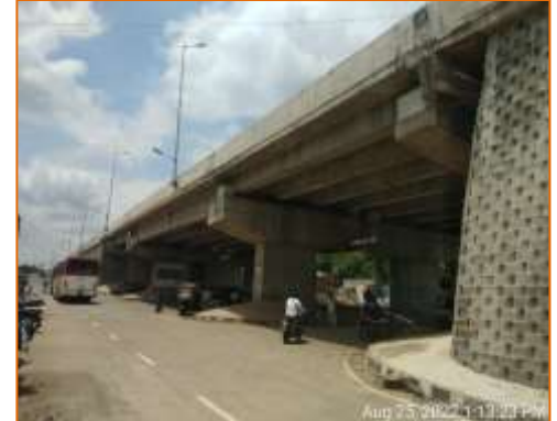
Side View of Flyover at km. 117.935 (RHS)
